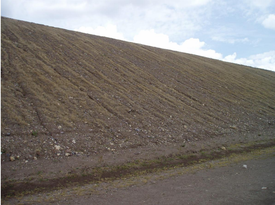
FIGURE 4-17: GRASS COVERING SLOPE OF DYKE OF RESIDUE DISPOSAL AREA.
