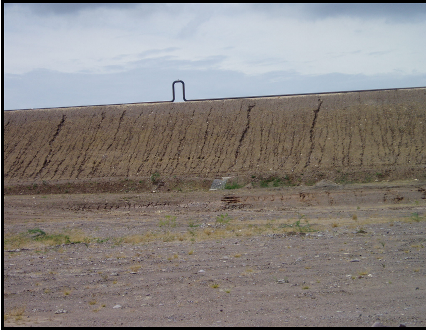
Figure 9: PHOTO OF AN RDA DYKE
