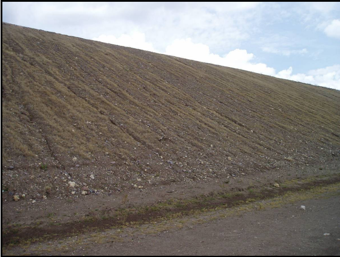
Figure 64: GRASS COVERING SLOPE OF DYKE OF RESIDUE DISPOSAL AREA.
