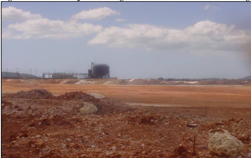
Figure 1-8: Bauxite Rejects in Foreground with Paste Thickener in Background
