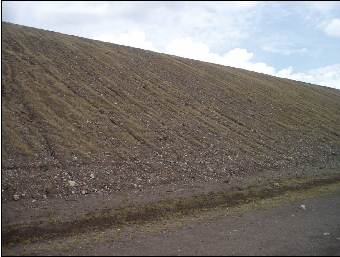
Figure 2-25: GRASS COVERING SLOPE OF DYKE OF RESIDUE DISPOSAL AREA.
