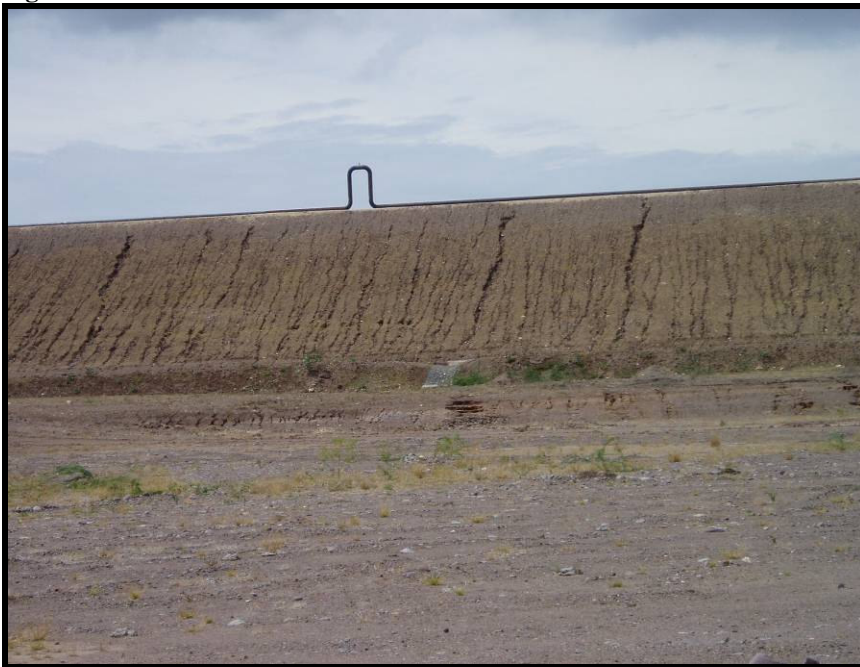
Figure 2-4: PHOTO OF AN RDA DYKE
