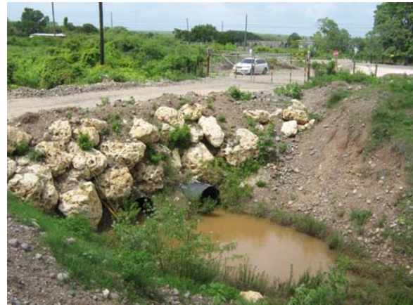
Plate 21: Drainage Canal running north to south of the RSA complex
