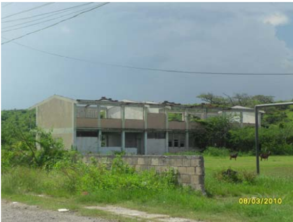
Plate 19: Dis-used School Building south of RSA complex
