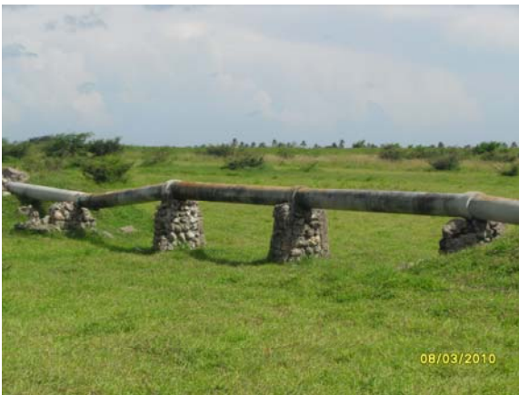
Plate 15: Appears to be a decommissioned pipe outlet (N17° 52.630' W77° 15.426')
