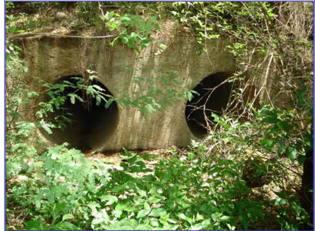
Figure 7: Culverts at the Old Harbour Bypass Road in the depression
