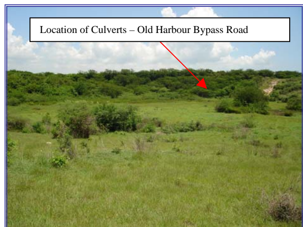
Figure 5b: Location of culverts at the Old Harbour Bypass Road in the depression
