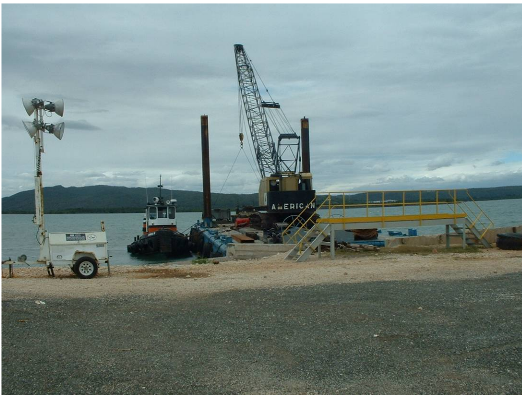
PLATE 2-3: BARGE DOCKED AT PROPOSED SITE FOR TEMPORARY UNLOADING DOCK
