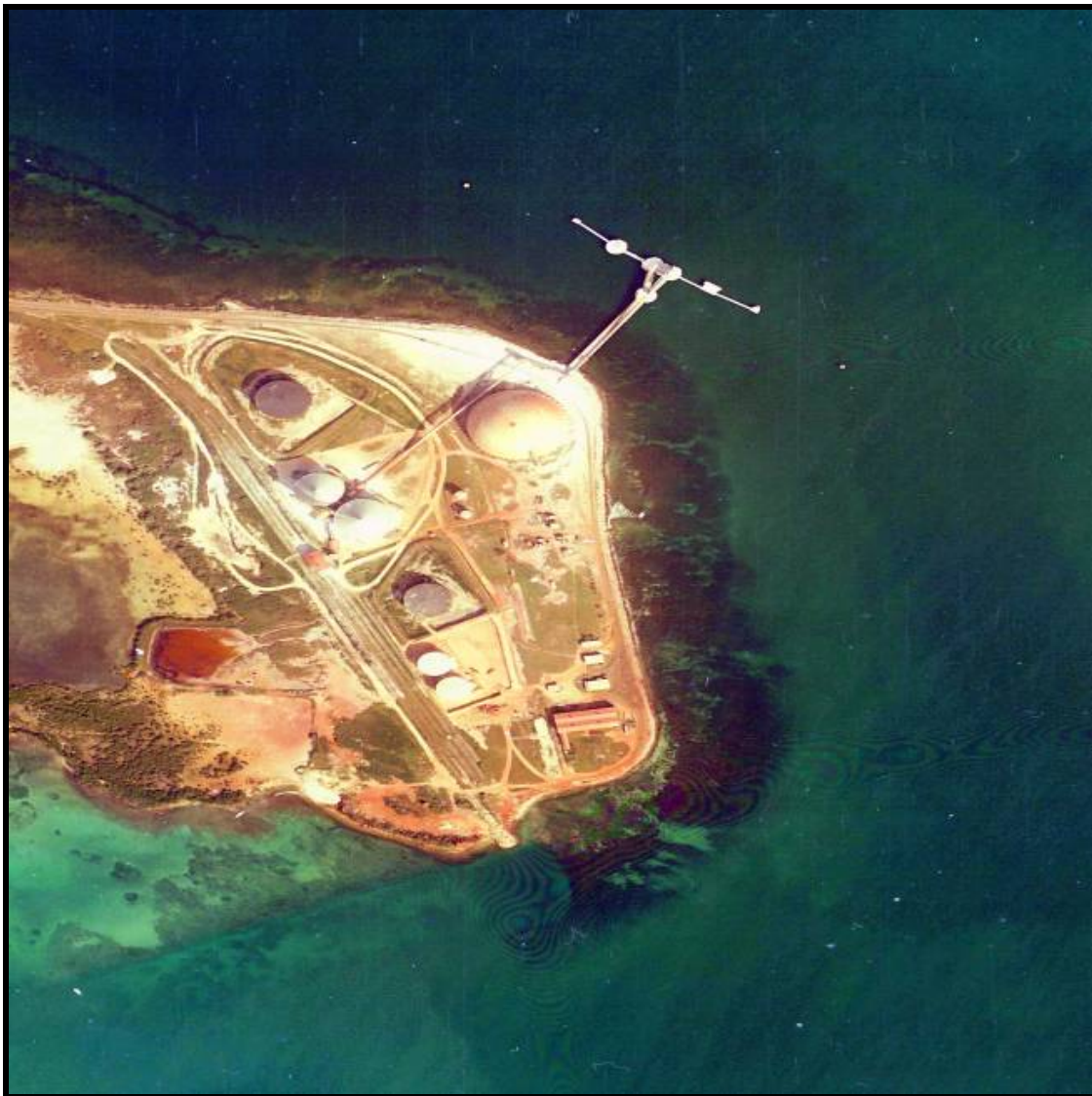
PLATE 4-17: T-SHAPED PILE PER AT JAMALCO ROCKY POINT PORT
