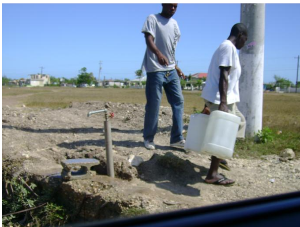
Community Water supply
