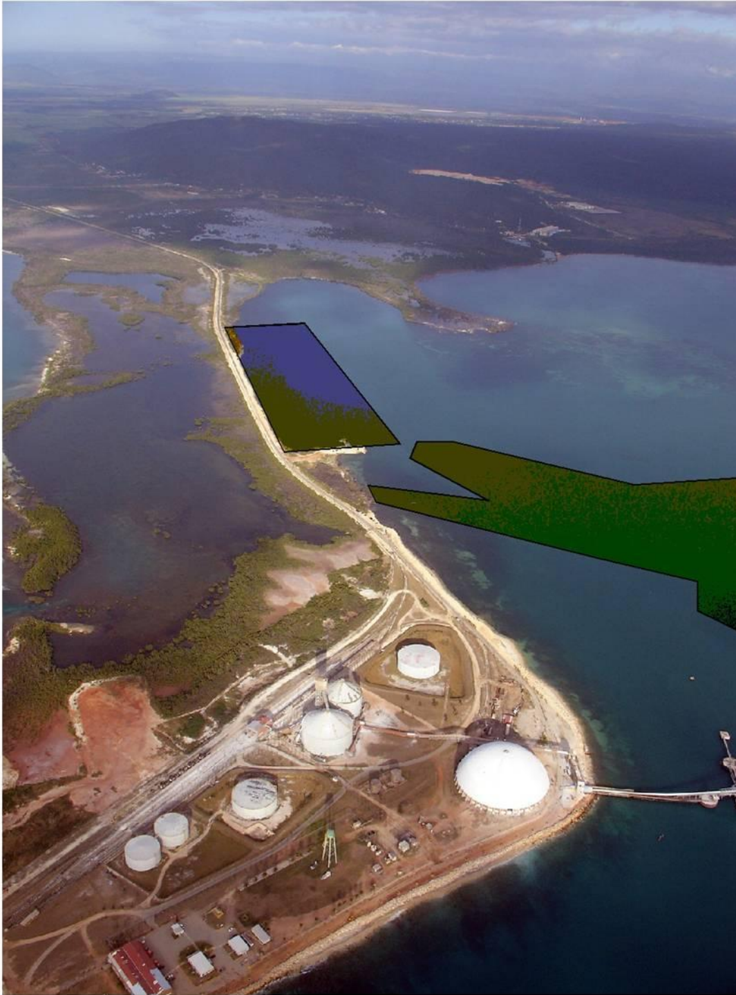
Plate 5-16: RINKER Development Site and Study Area [Overlain on oblique imagery - boundaries not to scale]
