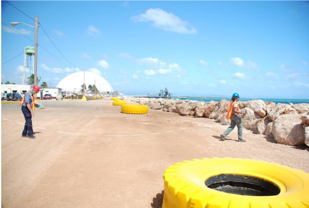
Plate 5-9: MGU personnel measuring inundation distances. The riprap on the right is of new, larger boulders replacing material that was moved across the parking area by hurricane Dean. (Photo taken 12/02/08)
