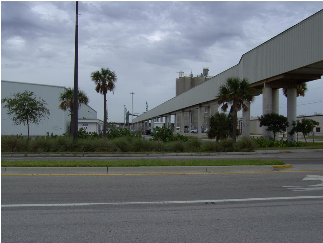
Plate 2-3: Typical Covered & Elevated Conveyor [Port Canaveral - USA]
