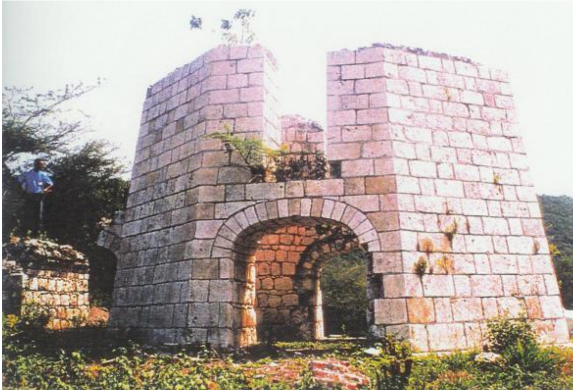
Plate 5-3: Old Cut Stone building off Salt River Road
