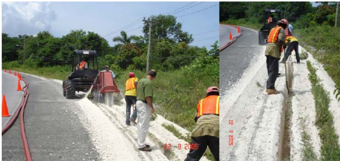
Figure 2-16: Trencher in Operation
