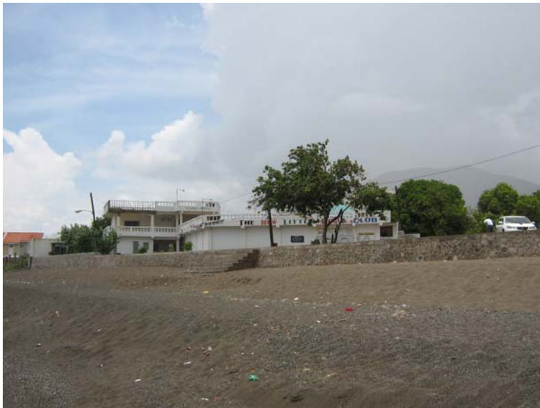
Plate 5-2: View from the shoreline (Looking northwest)
