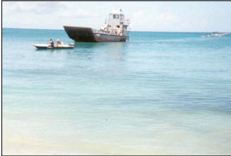
Plate 2-4: Illustration of Installation Using a Landing Craft
