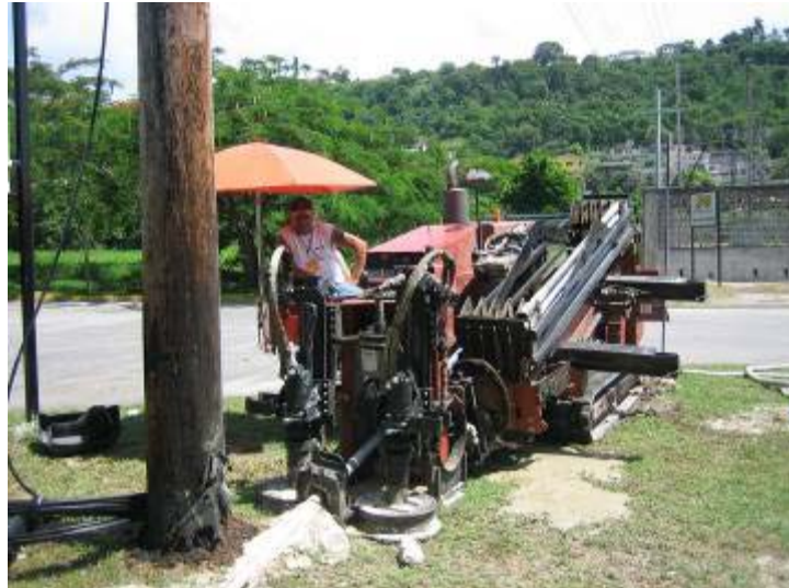
Plate 2-1: Horizontal Direction Drill - Ditch Witch JT2720
