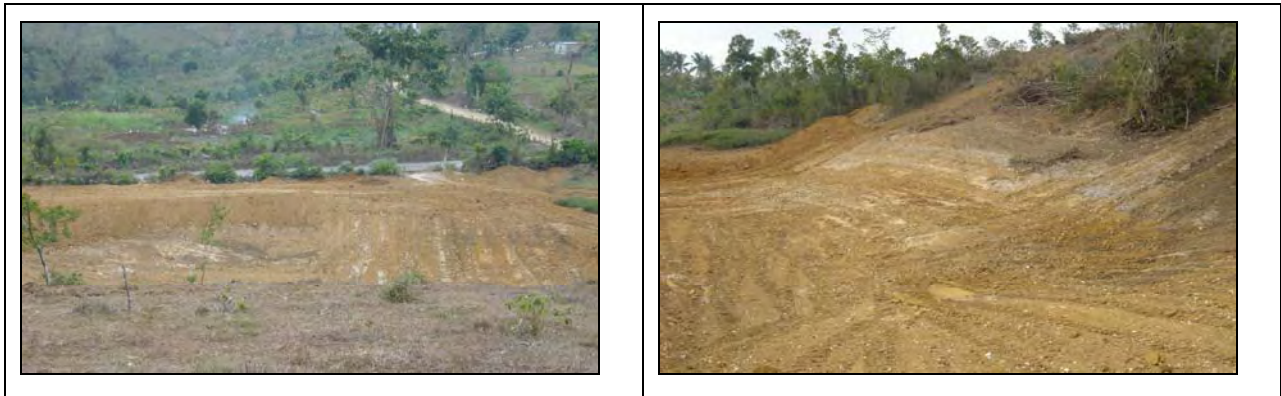
Figure 23 Photos of the Pond on the Property
