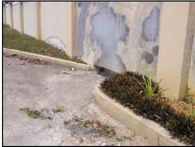
a/ Drain from main road to the site
