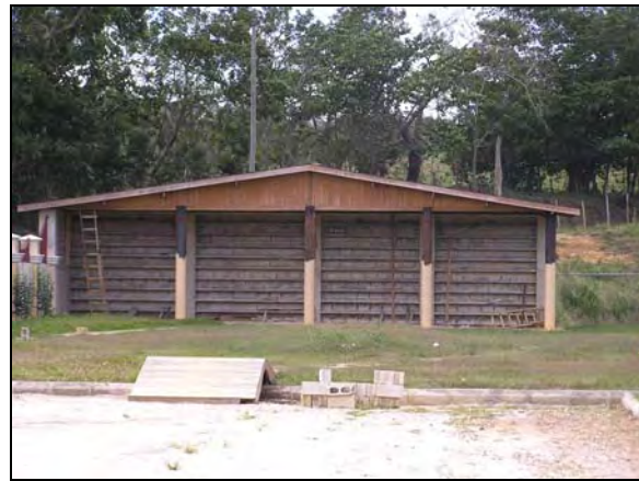
b/ Structure on south-western corner of property.
