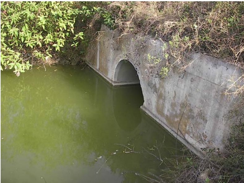
Figure 5: Submerged outlet of culvert 3
