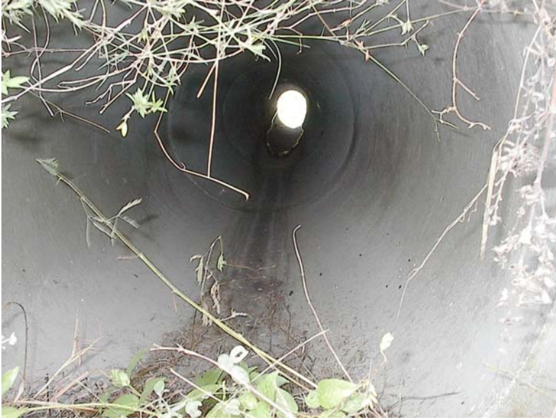
Figure 4: Inlet of culvert 3, 900mm in diameter
