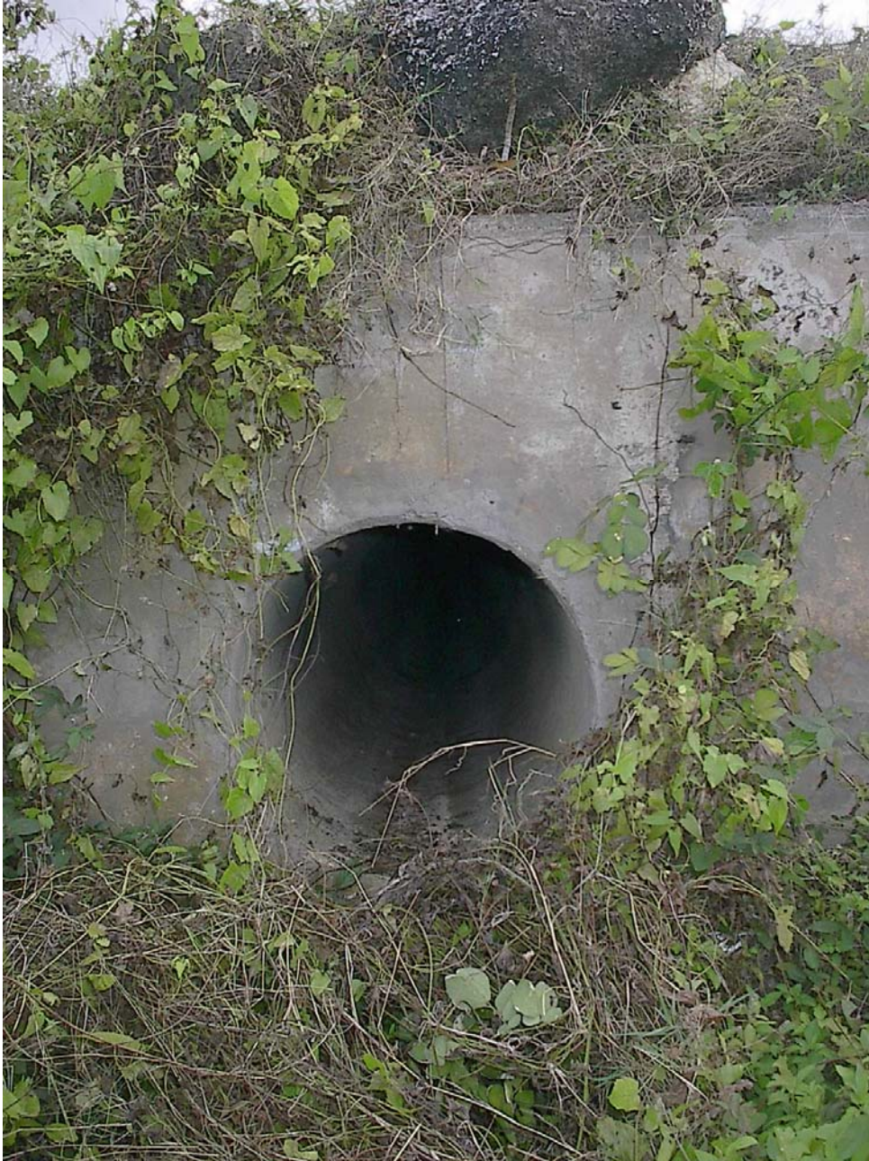
Figure 3: Outlet of Culvert 2 (600mm in diameter) - to West Cove
