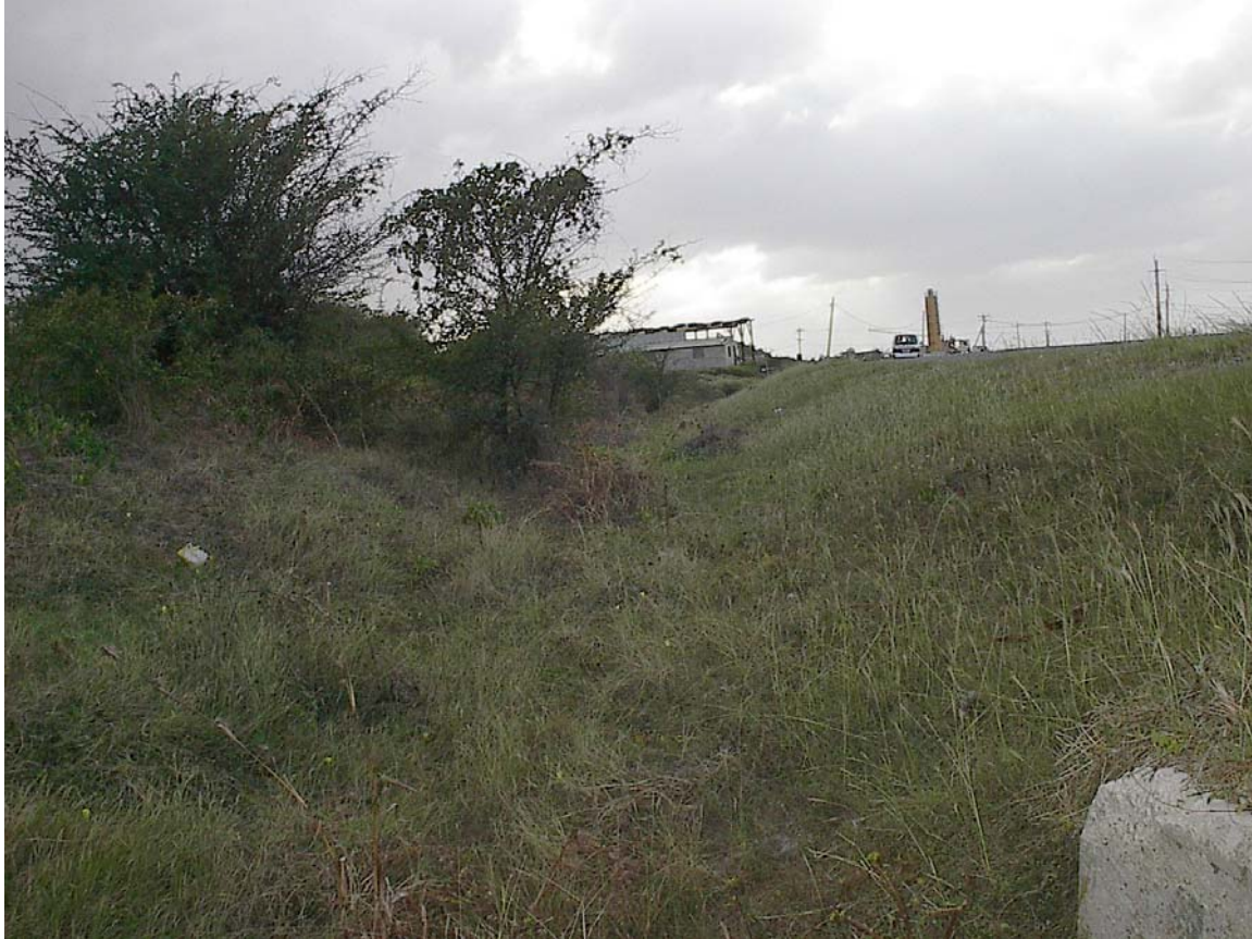
Figure 2: Inlet of Culvert 1 (600mm in diameter, East of Bosung yard)
