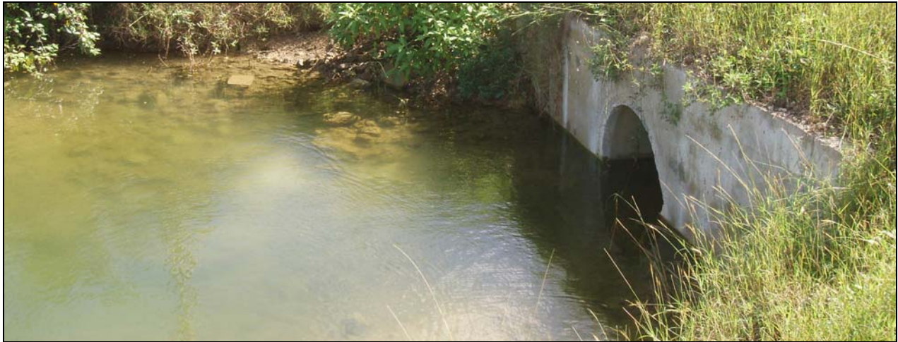
Figure 17 Culvert on property
