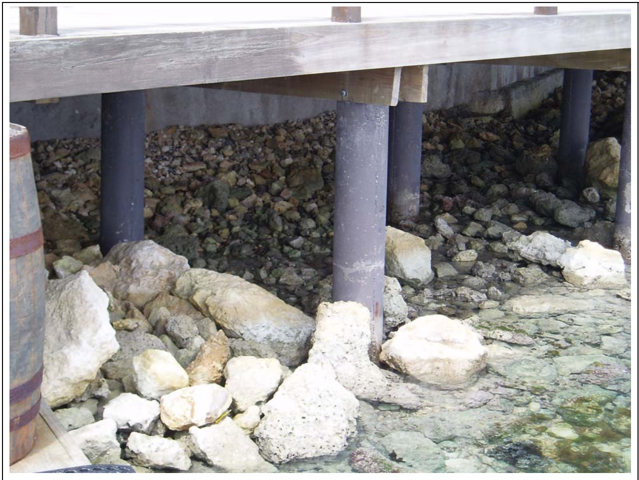
Figure 5 Photo of boardwalk showing pvc pilings
