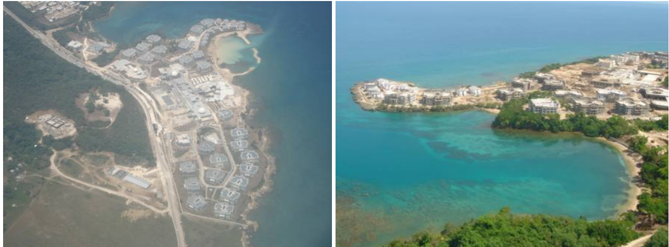
Figure 1.2 Man-made beach on the northern resort shoreline (left) and natural beach cove on the southern resort shoreline (right)
