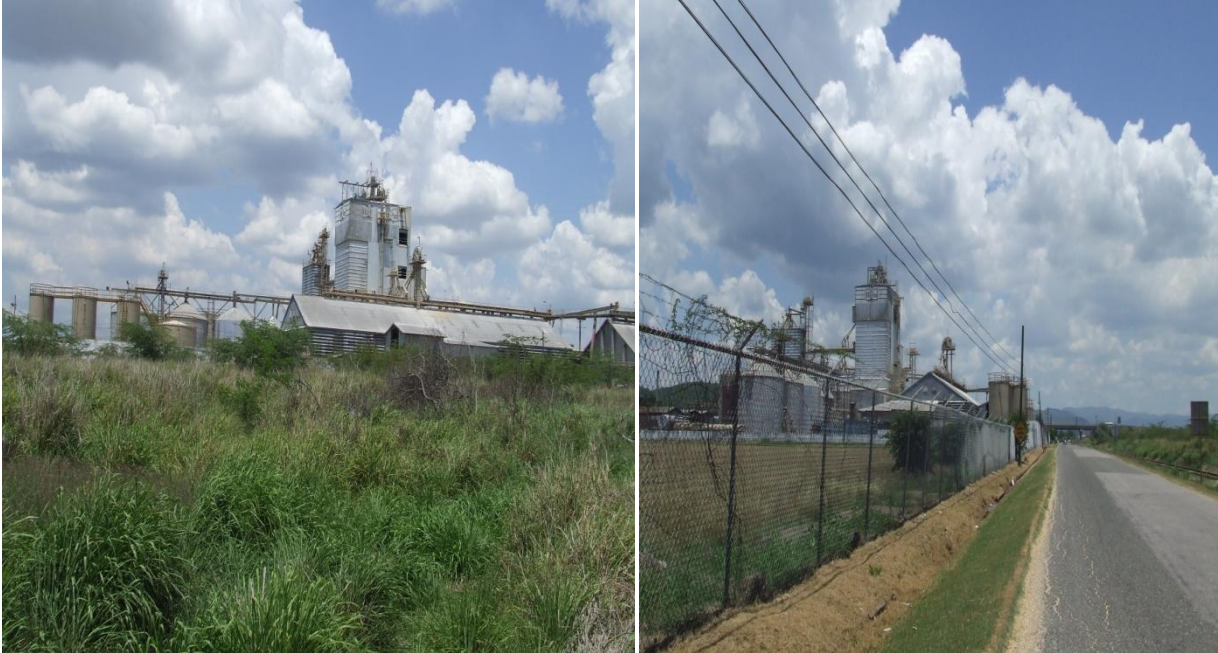
Figure 12: HIPRO FEEDS seen from the plant site and road way alongside the railroad
