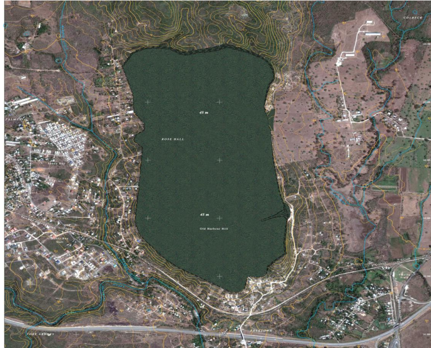
Figure 43: Aerial view of deposit area after limestone quarrying.
