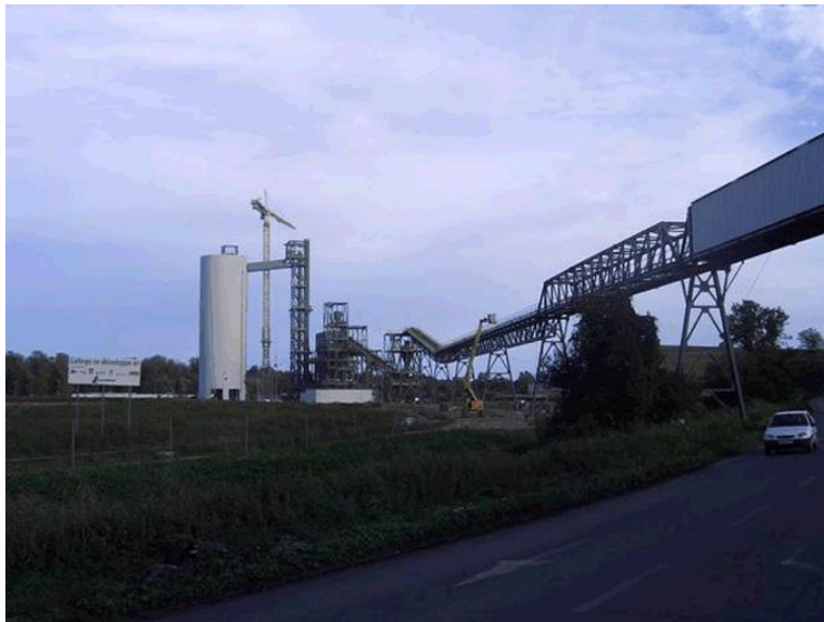
Figure 30: Photo of typical conveyor crossing the highway
