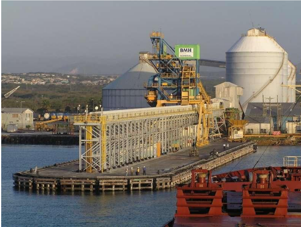
Figure 27: Port Esquivel – Port Facility
