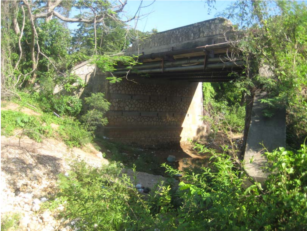
Figure 3-5. Box Culvert under Old Harbour main road.
