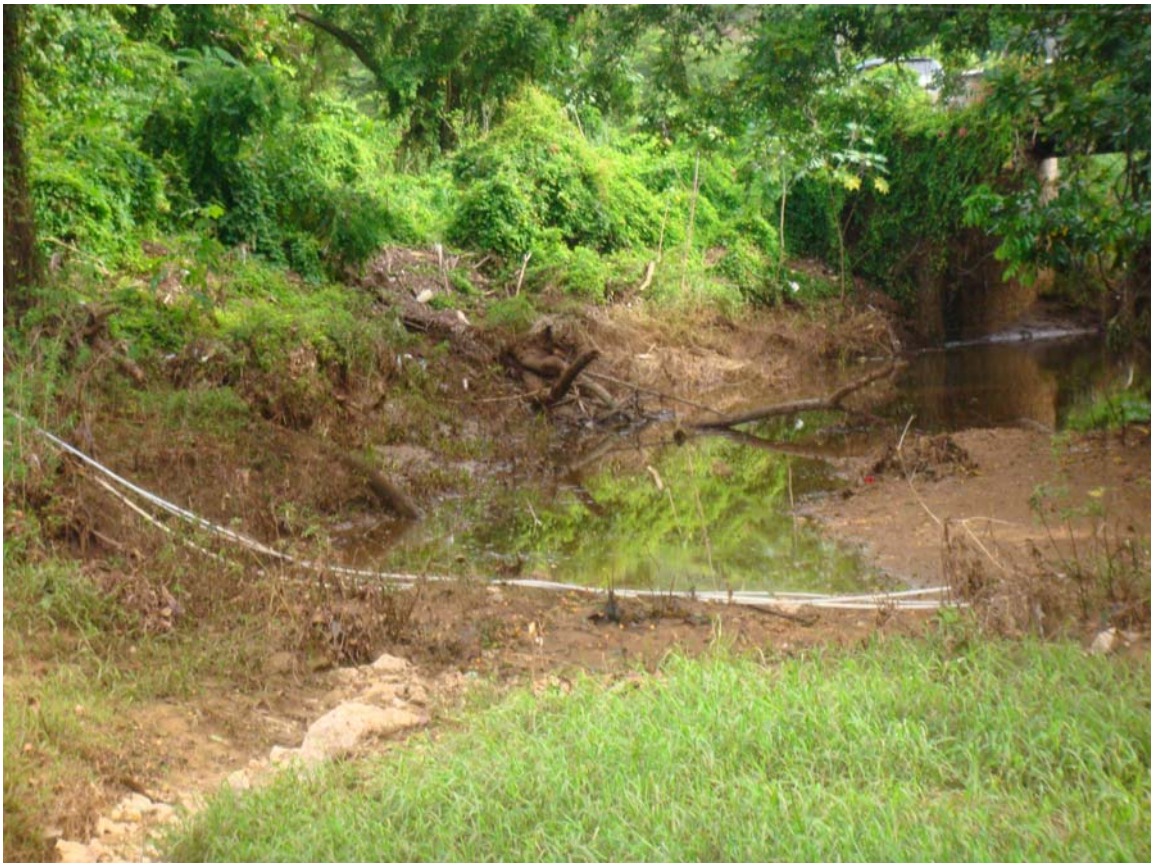
Plate 3.1. Picture shows Clarendon gully looking upstream toward culvert under Highway 2000
