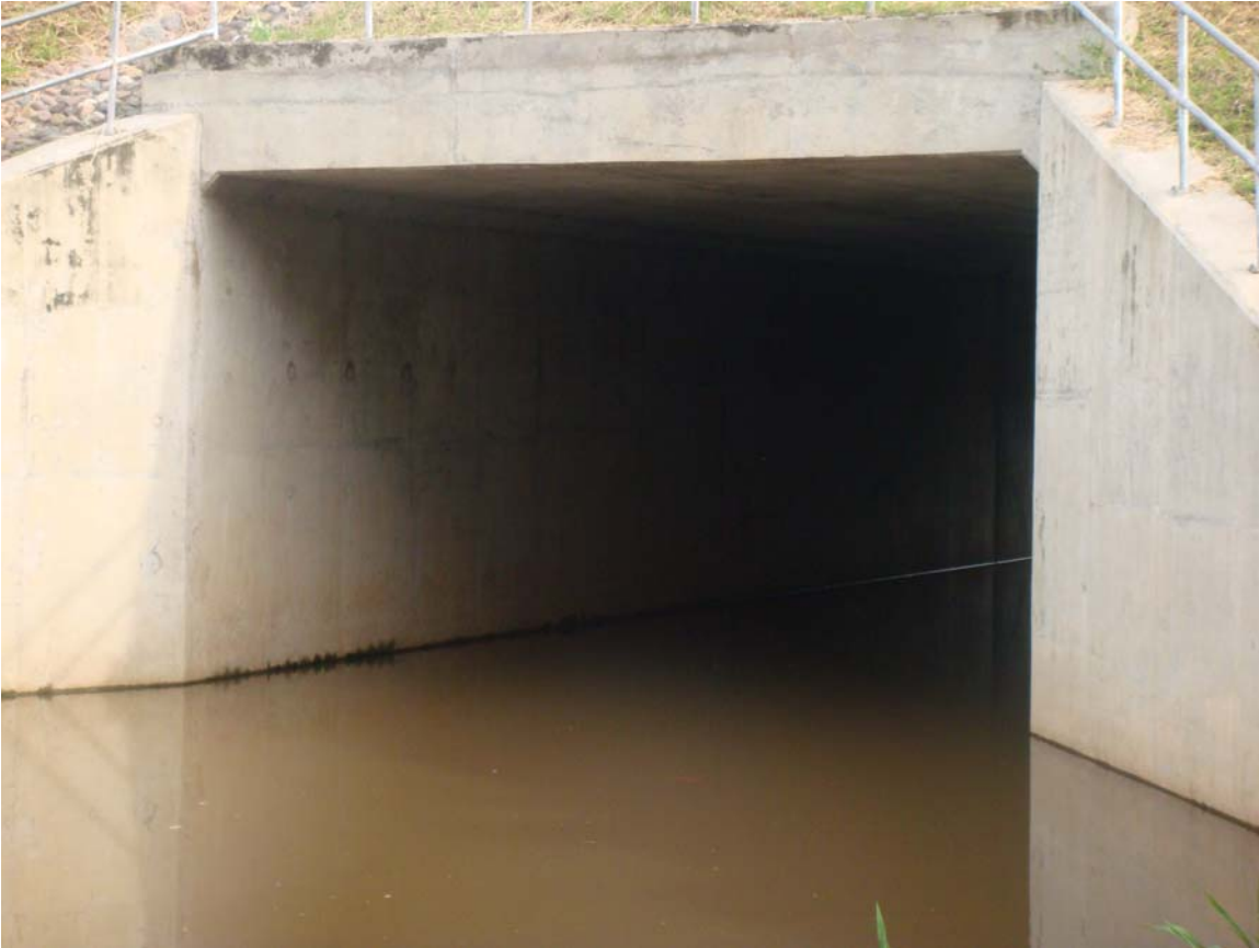
Plate 3.2. Concrete culvert under Highway 2000 is the channel for the Clarendon gully.
