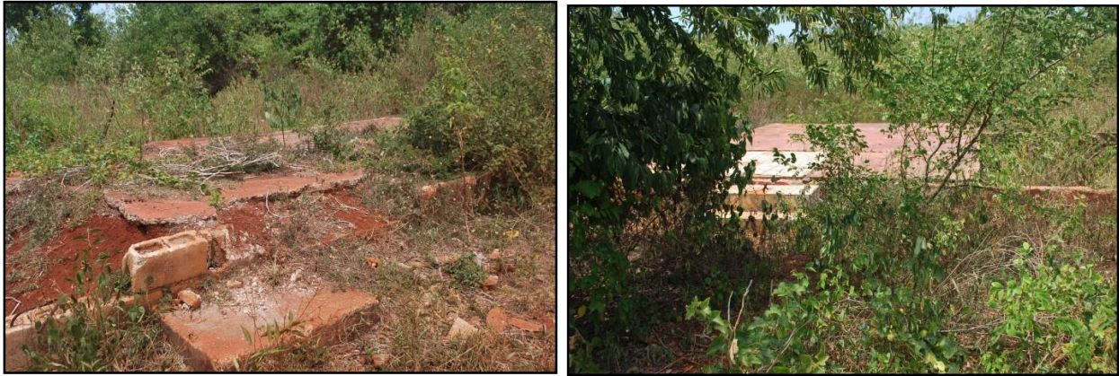
Plate 4-10 Foundations of recently demolished structures
