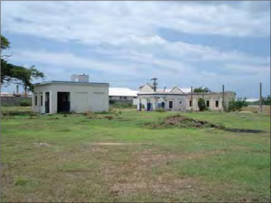
Plate 2 Existing building on site: Remnants from the NWC Treatment Plant
