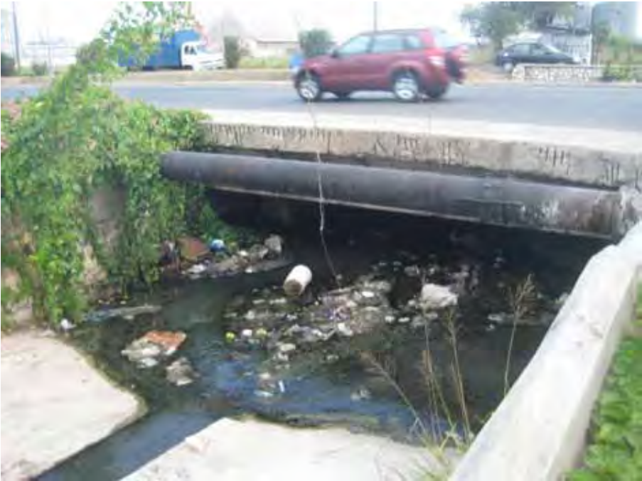
Plate 6 Box Culvert under Marcus Garvey Drive.
