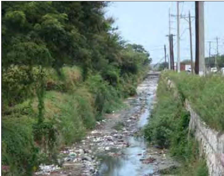
Plate 7 View of the Tivoli Gully (looking south) from Producers Road
