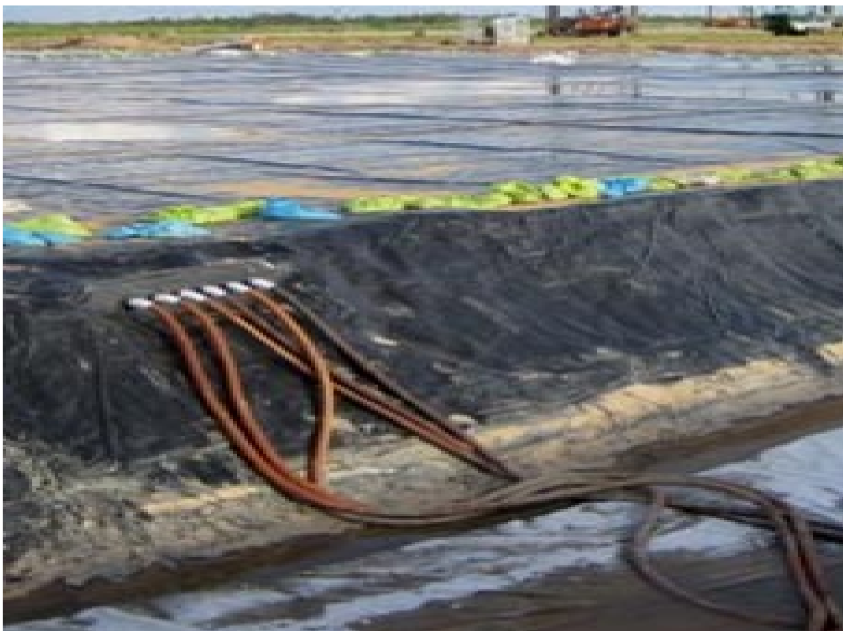
Fig.21 The surcharge method of compacting newly placed granular reclamation fill
