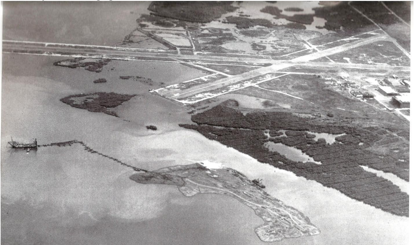
Fig 8 above is a 1955 aerial photo showing a cutter suction dredger (CSD) operating in the Palisadoes wetlands at the start of construction of Palisadoes Airport, which later developed into becoming the present Norman Manly International Airport, NMIA. Over eight million cubic yds of seabed material was dredged to create the 310 acres of new land, using this flat bottom, shallow draught CSD and the “pump ashore “ method of reclamation.
