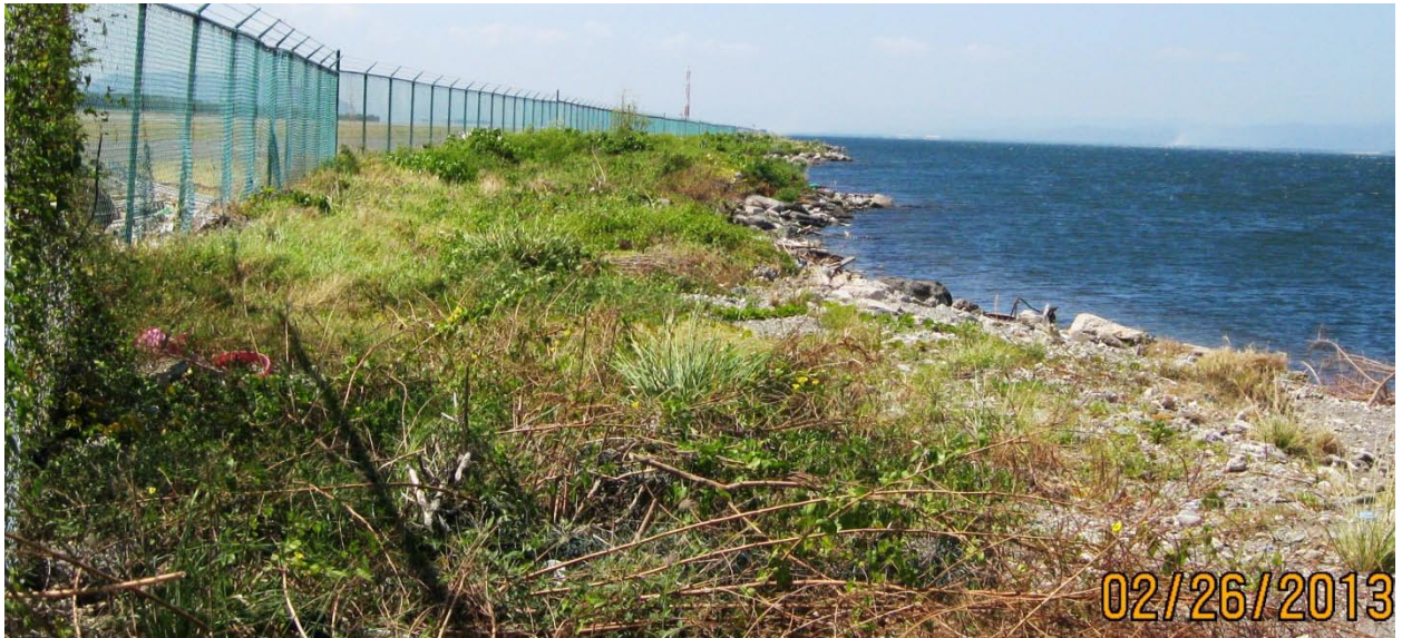
Fig. 3 Photo looking westwards along the north edge of the existing runway. This portion of the runway is to be widened by 15m, Reclamation area B in the above Fig.2
