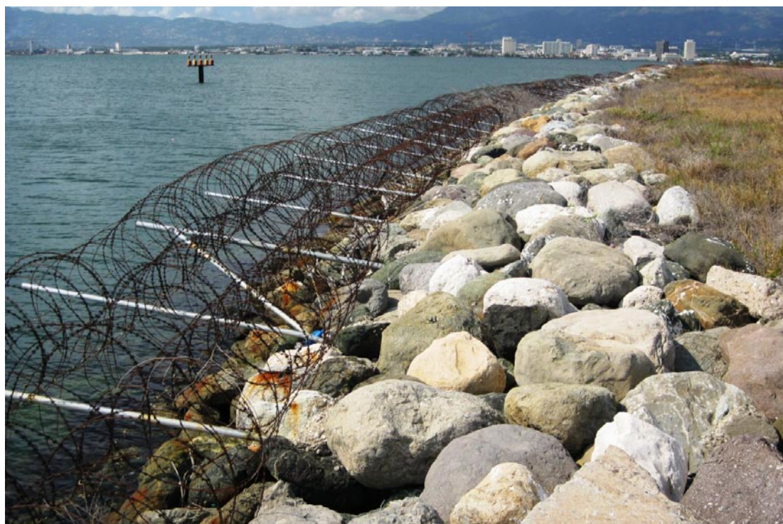
Fig.20 Photo looking north along the tip of the runway showing existing slope protection
