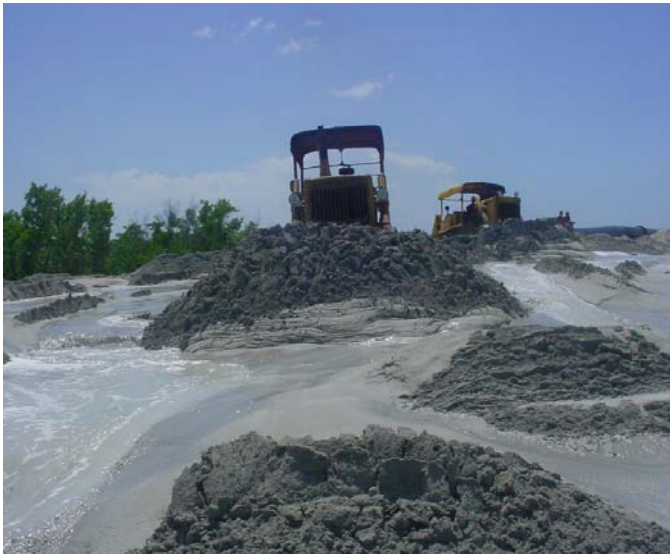
Pictures 25 and 26. Spreading of fill material for the conformation of the dune and beach profile.
