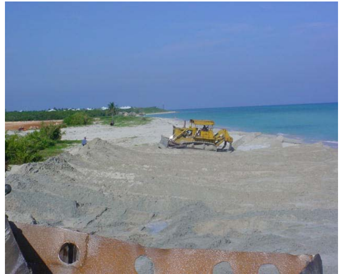
Pictures 25 and 26. Spreading of fill material for the conformation of the dune and beach profile.
