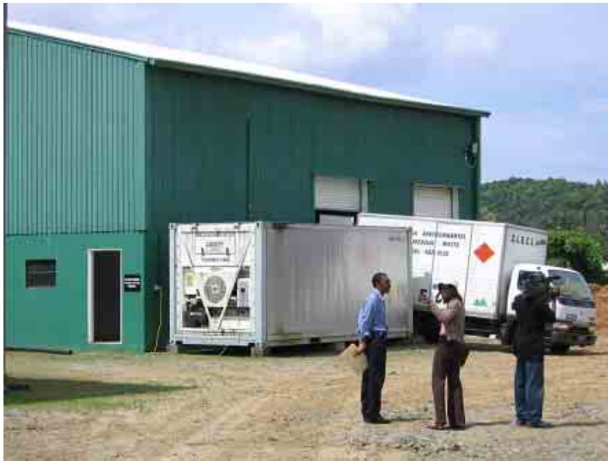
Plate 4.8 Example of the type of building for the Medical Waste Treatment Facility
