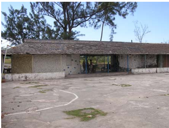
Figure 7 Structures slated for Demolition
