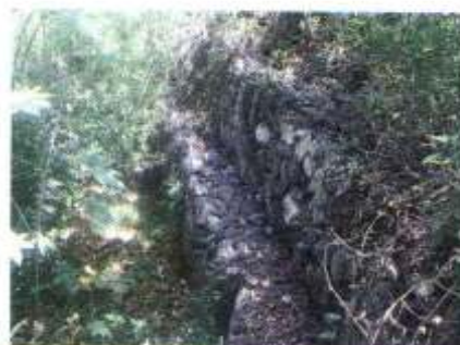
Figure 5: Gabion baskets
