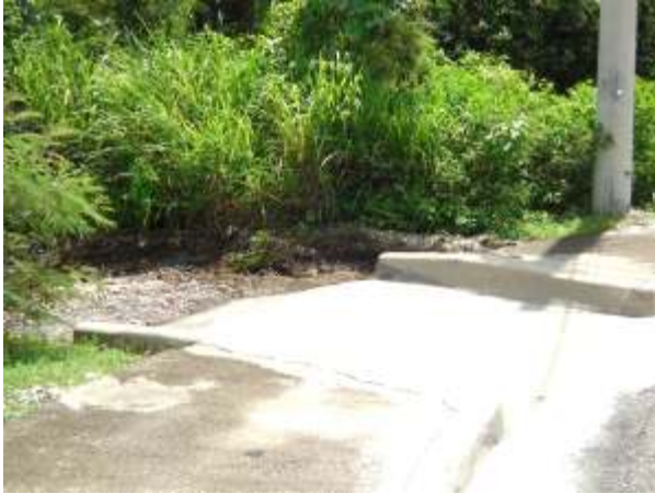
Plates 6.4 A and B: Spillway and grided cross drain along the access road
