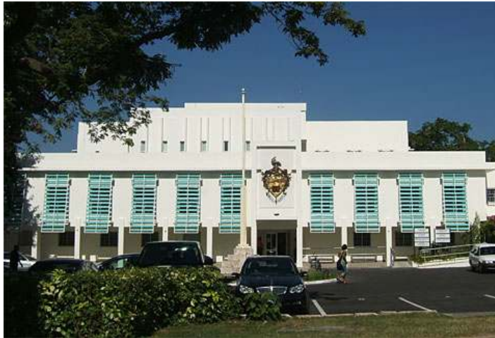
Plate 6.6: The Annex building at the University of West Indies, Mona
