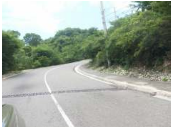
Plates 6.4 A and B: Spillway and grided cross drain along the access road
