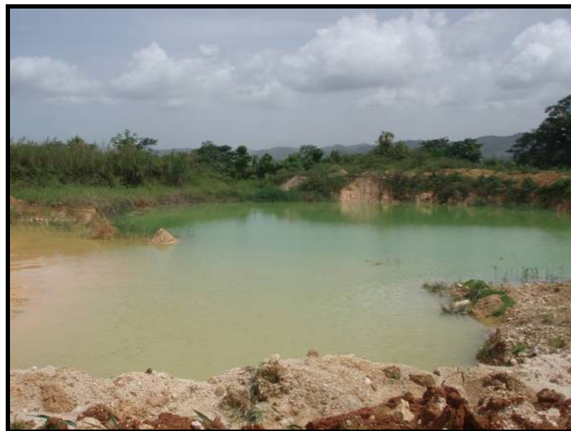
Plate 5-4: Pond with Wastewater from the crusher (wastewater re-circulated)
