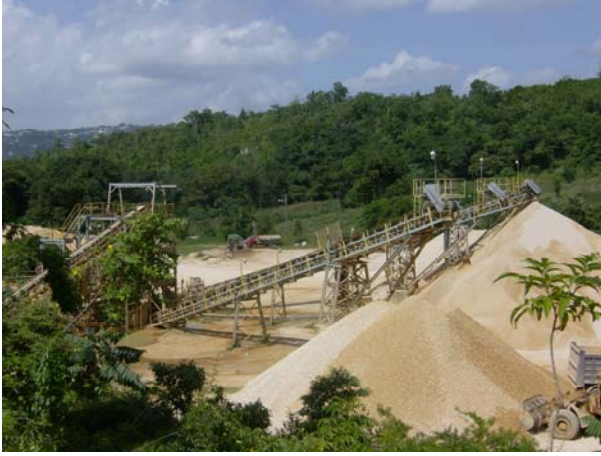
Figure 9-6: Stockpile Area [Main area for placement of new lime kiln]
