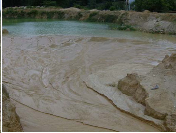
Plate 9-20: Pond 5 - Sand material at entrance collected and stockpiled
