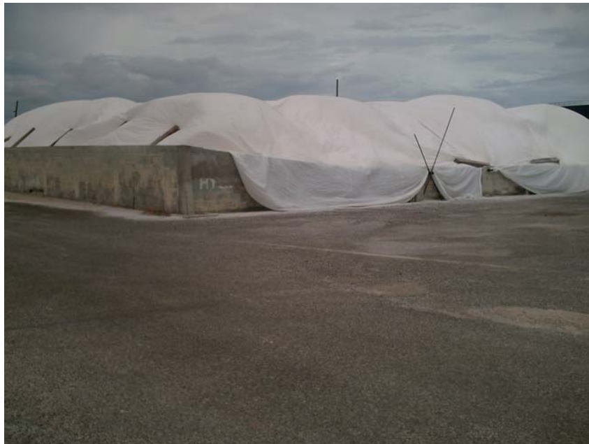
Plate 2-4: Bunded Area for Hydrate [Note: Fuel will be covered with tarpaulin similar to that used here]
