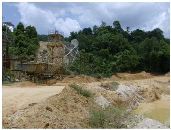
Plate 9-15: Crusher and associated equipment
