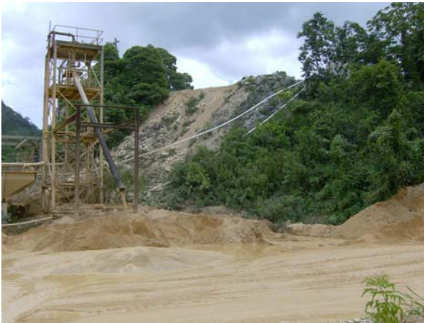
Plate 9-13: Aggregate wash material wastewater pipe near crusher
