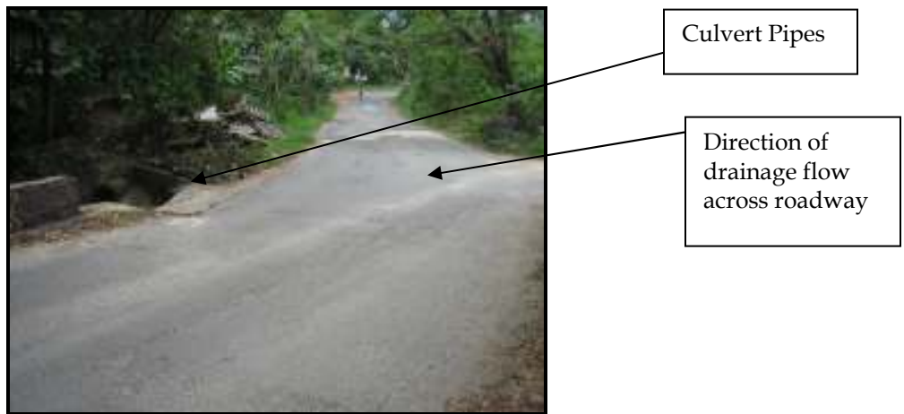
Plate 17: Looking north on Mannings Hill Road the Shingle Hut Gully is culverted across the road.
