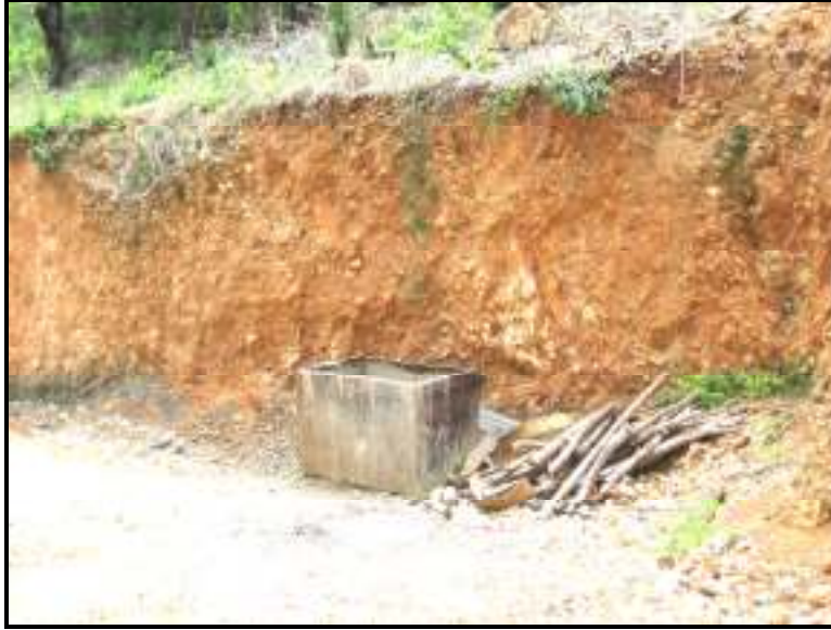
Plate 6: Highly weathered and fragmented limestone (cobble size Limestone) exposed on an excavated cut adjacent to the project site
