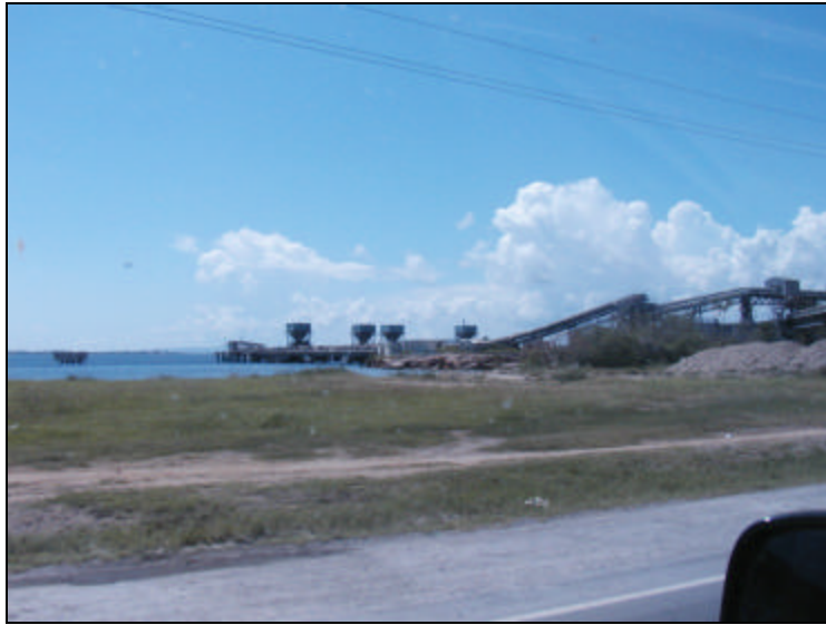
Plate 4.2 Factory and Shipping Facilities Looking Northwest
