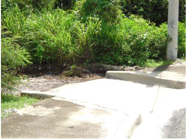
Plates 6.4 A and B: Spillway and gridded cross drain along the access road
