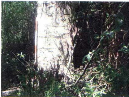
Figure 4: Cut stone structure encountered in the large depression
