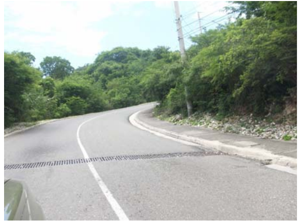
Plates 6.4 A and B: Spillway and gridded cross drain along the access road
