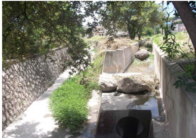
Plate 7.1: The Pines of Karachi drain as it enters the larger paved drain down stream
