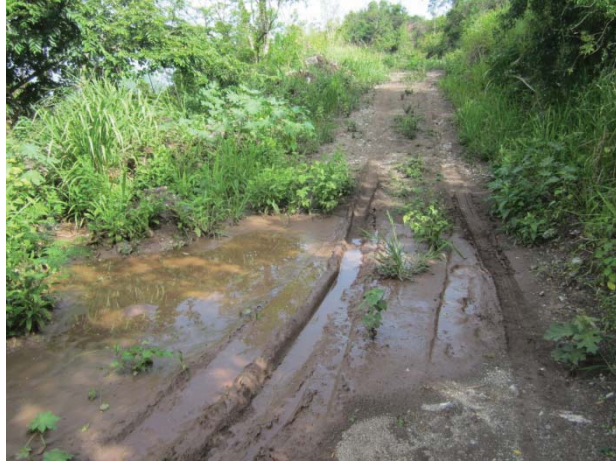
Plate 2.5 Condition of local road after passage of Tropical Storm Chantal (2013);
