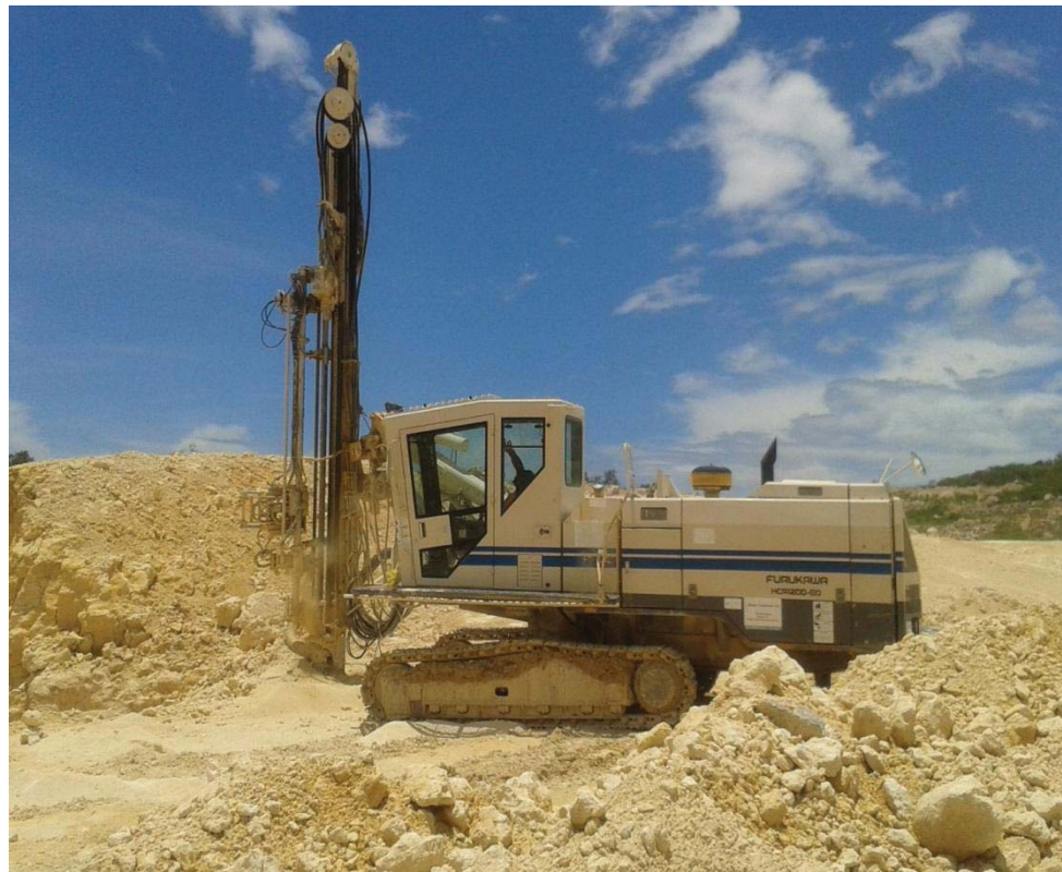
Plate 5.1 Production holes being drilled for blasting using the Ingersoll Rand drill
