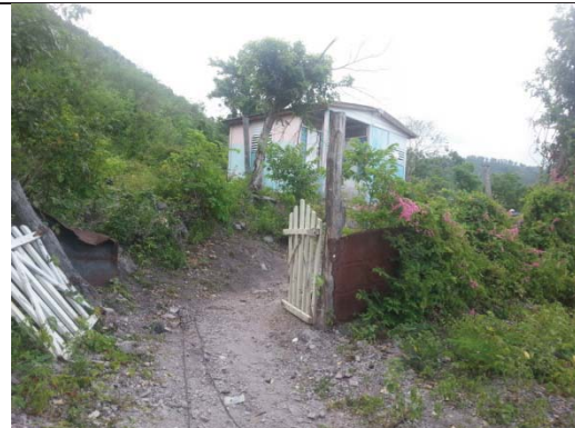
Plate 2.2 Residence with wooden structure
