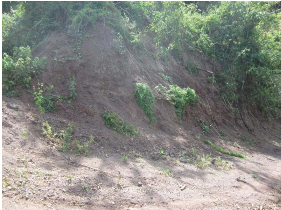
Plate 6.5 Third landslide located during site visit (#524)
