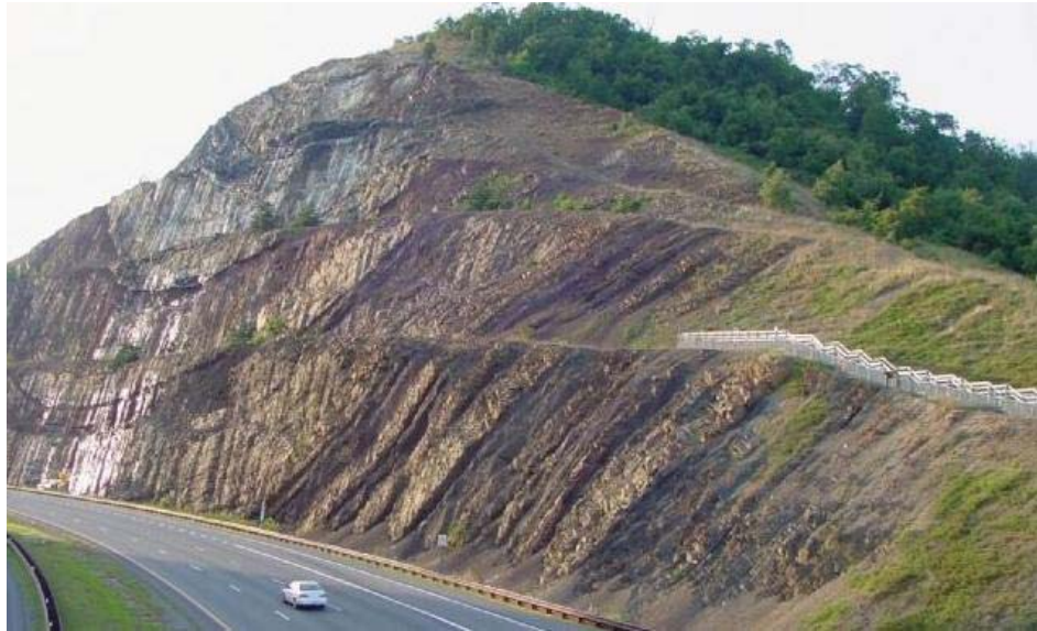
Plate 9.3 Bench trail cut on face of steep slope
