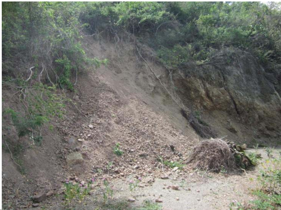
Plate 6.4 Second landslide identified during field reconnaissance (#520)
