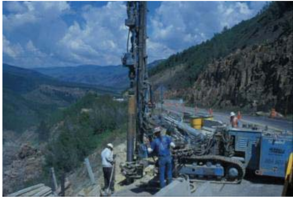
Plate 9.2 Installation of metal soil nails at edge of slope
