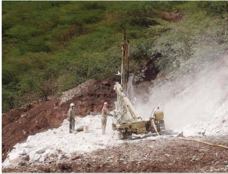
Plate 2. Production holes being drilled for blasting using the Ingersoll Rand drill
