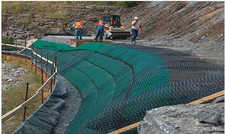
Plate 9.5 Geogrids being placed on face of slope
