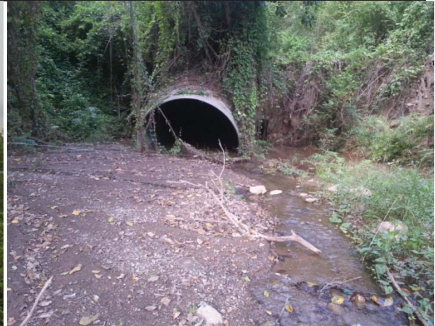
Plate 2.8 9" corrugated culvert which conducts Bull Park River flows under local road;
