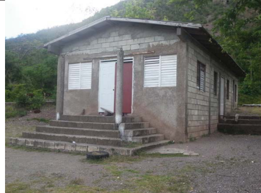
Plate 2.4 Structure constructed of concrete
