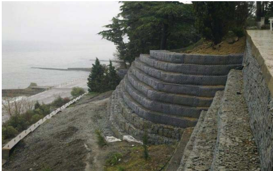
Plate 9. Gabion walls erected along face of steep slope
