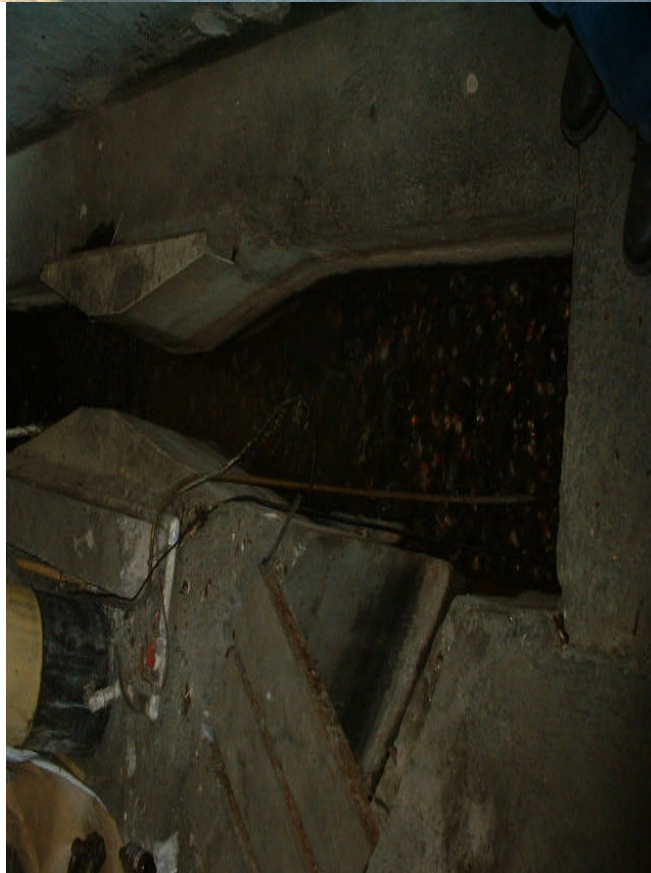
FIGURE 7-11: MONITORING STATION 3 (BREW HOUSE) WITH ASSOCIATED DRAIN
