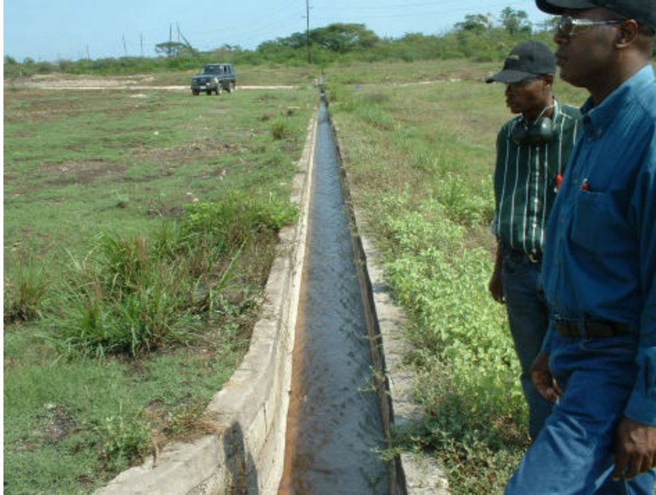
FIGURE 7-7: TYPICAL VEGETATION WITH EXISTING DRAIN
