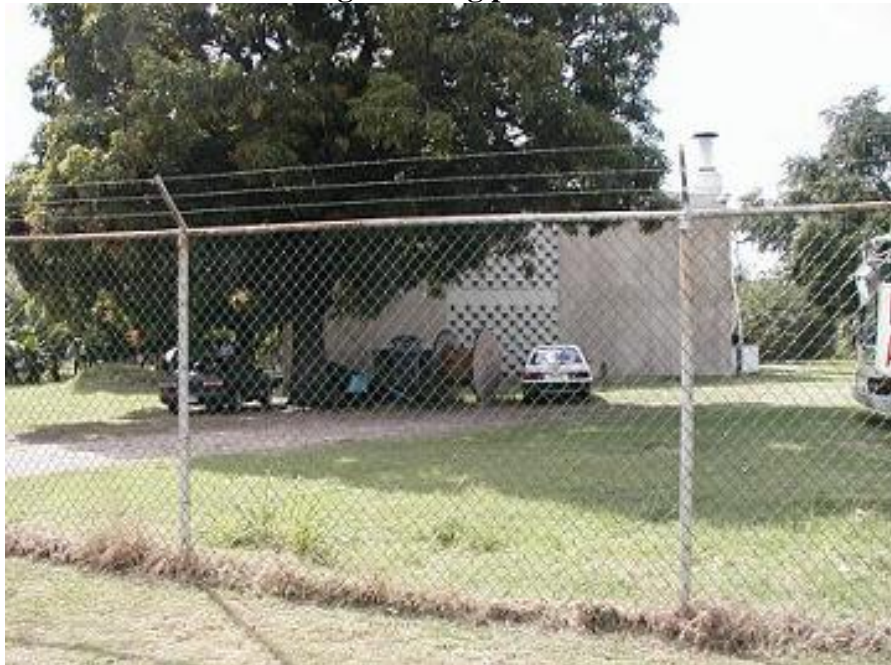
Figure 5.4 Site for new incinerator (in the foreground) adjacent to the standby power generating plant
