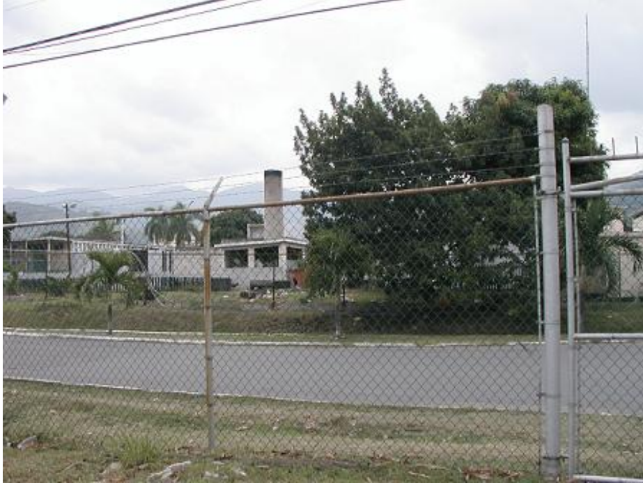
Figure 5.3- Picture taken from the site for the new incinerator showing the stack of the existing incinerator across the road
