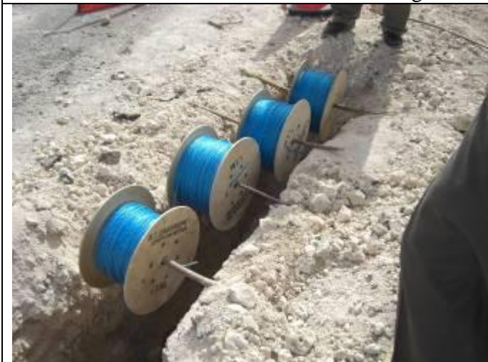
Laying ducts and installing draw rope
