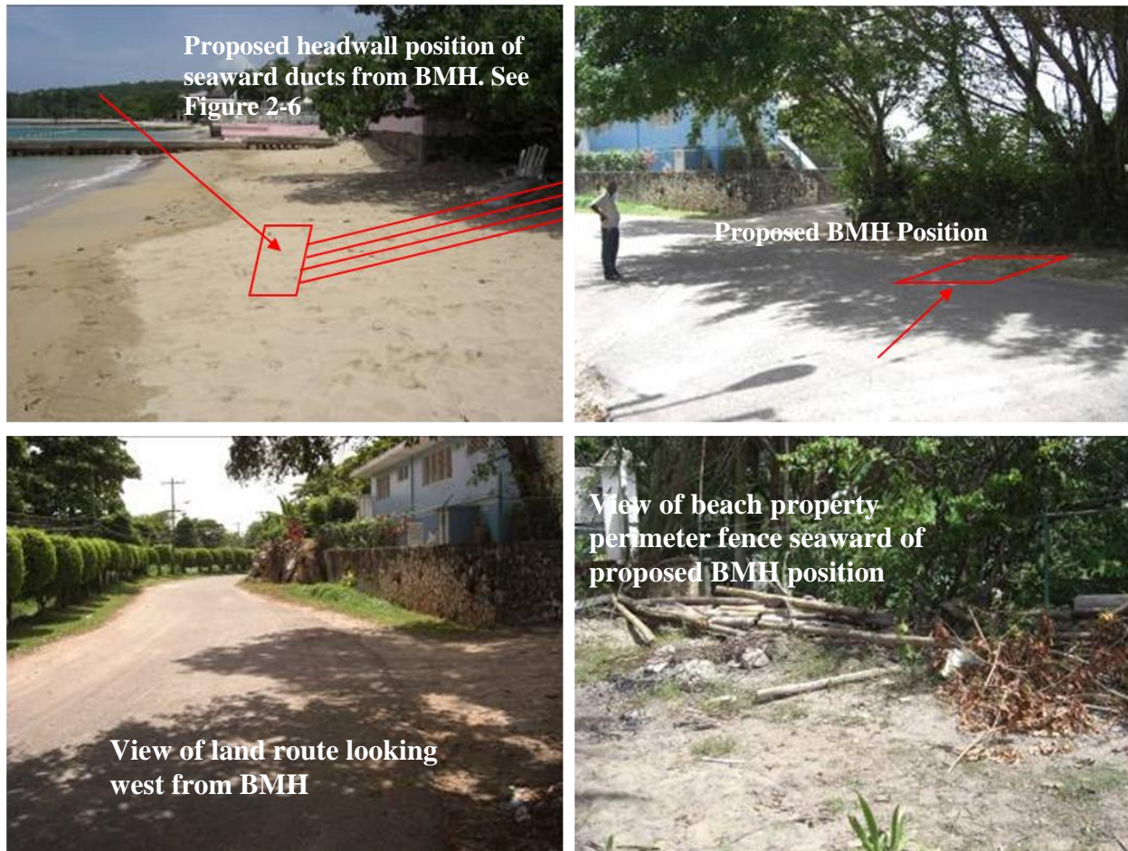
Plate 2-5: Beach Manhole Location View of beach property perimeter fence seaward of proposed BMH position
