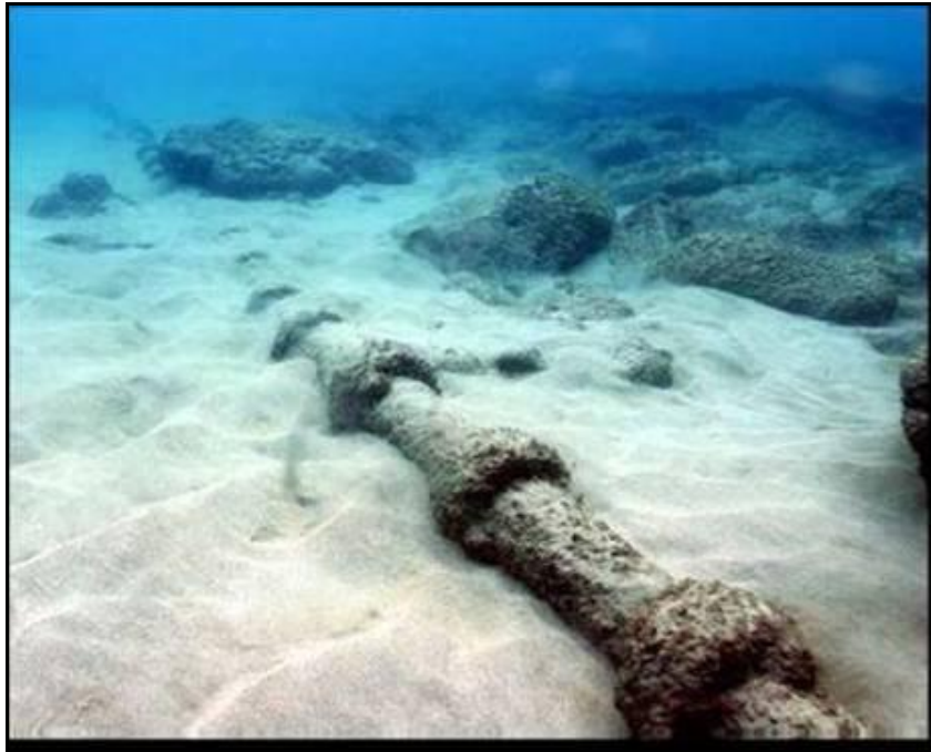
Plate 2-10: Articulated pipe protection with self-interlocking/split sleeve
