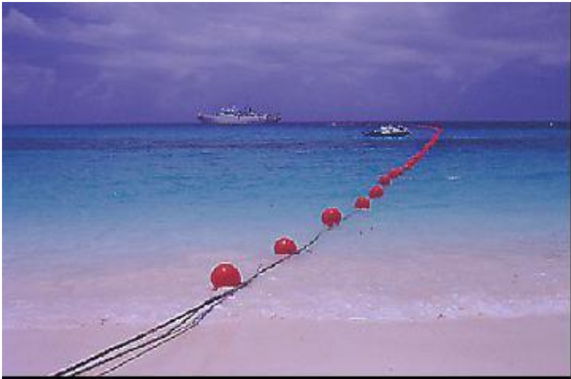
Plate 2-9: Floats affixed to cable during a cable installation
