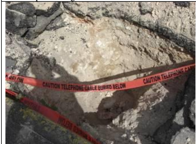
Test hole dug at planned manhole position
