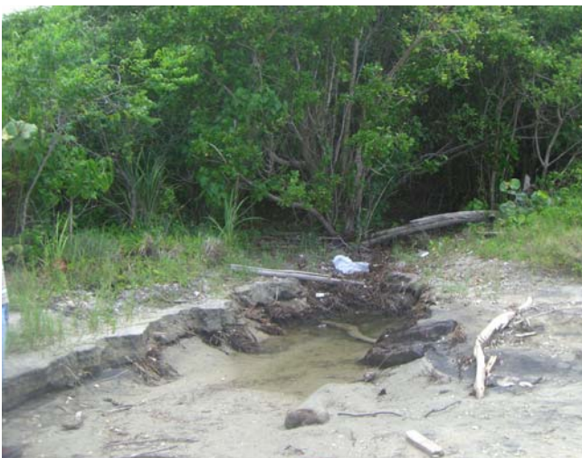
Plate 4-5: Erosion observed at northwest corner of site
