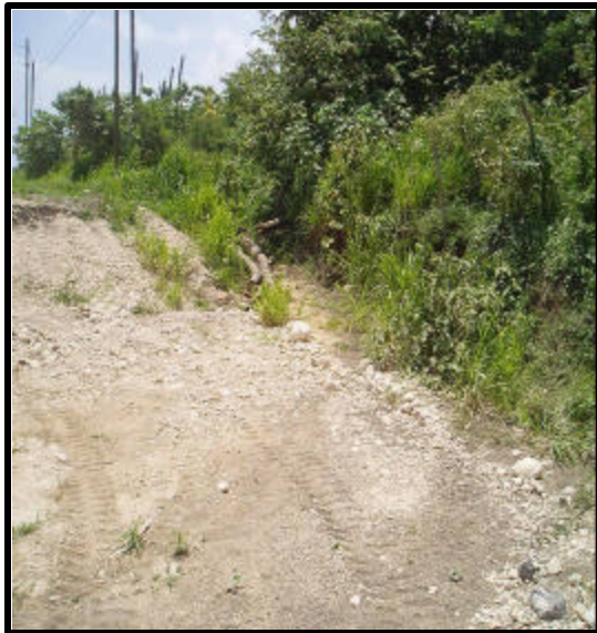
Plate 3.5: Richmond Estate Gully (Northern Exit)
