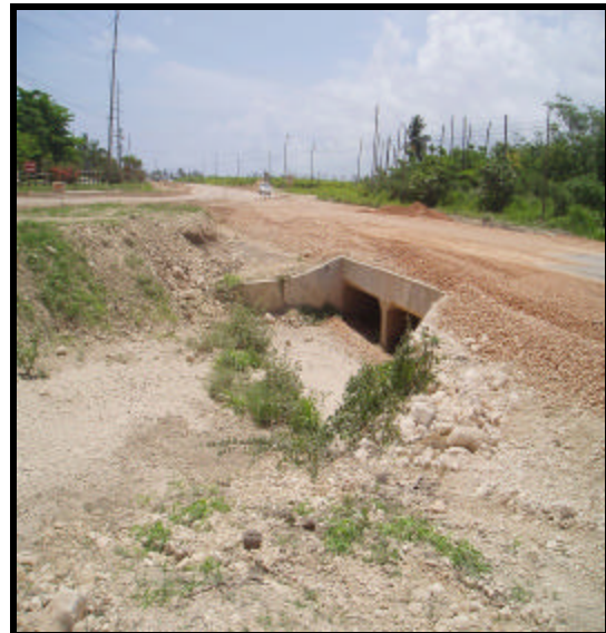
Plate 3.6: North Coast Highway Culvert for the Richmond Estate Gully
