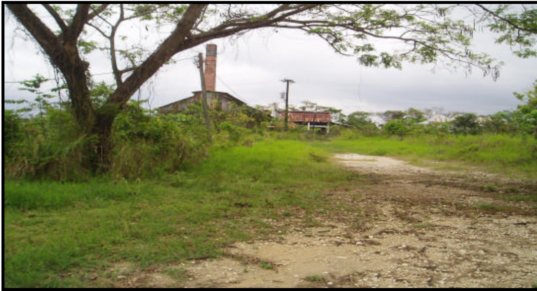
Plate 3.16: The ruin of the old Richmond, Llandoverly sugar factory
