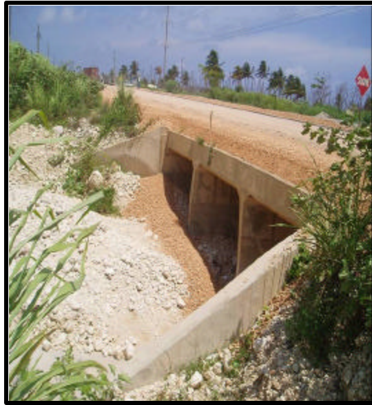
Plate 3.8: Stony River (Culvert on North Coast Highway)
