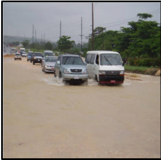
Plate 3.10: Flooding of North Coast Highway at Richmond Estate-Chukka Cove
