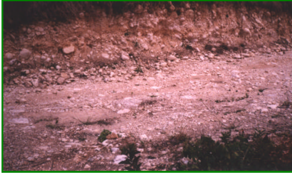
Plate 9: Cleared existing channel.
