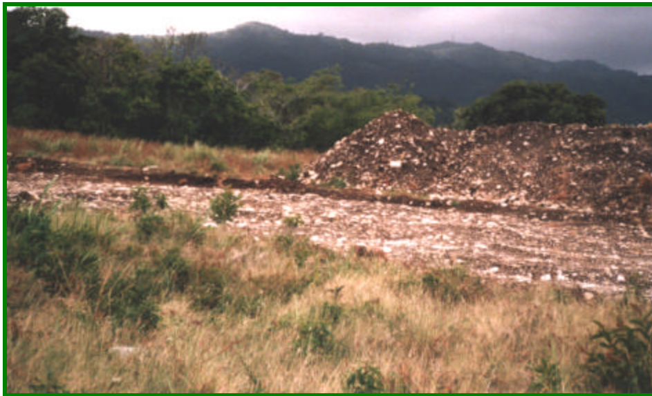
Plate 8: Gully that was cleared.
