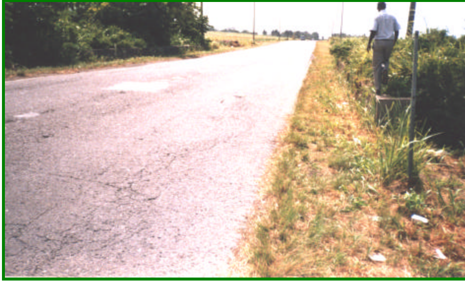
Plate 19: Drain running alongside North Coast Highway. (Property boundary is to right of photograph).
