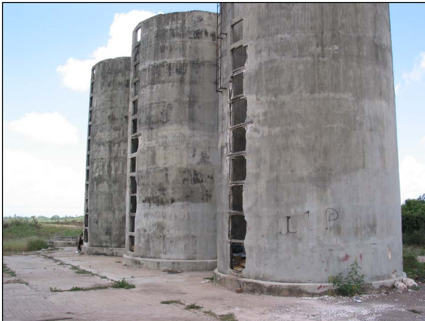
Plate 32. Abandoned silo used for burning waste.
