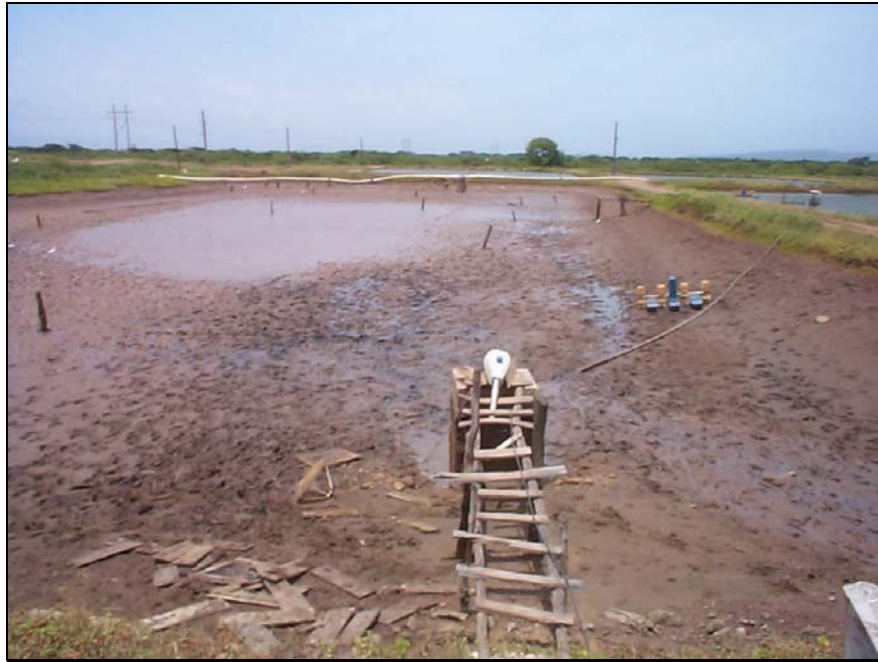
Plate 19. Drained shrimp pond showing concrete monk in foreground.
