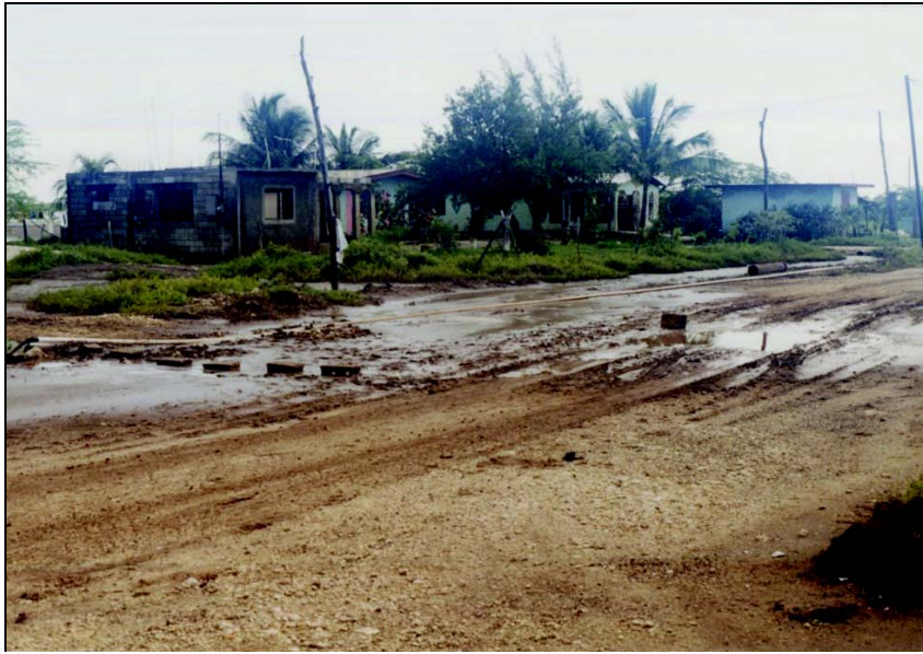
Plate 25. Homes along Thompson Pen Lane vulnerable to flooding.
