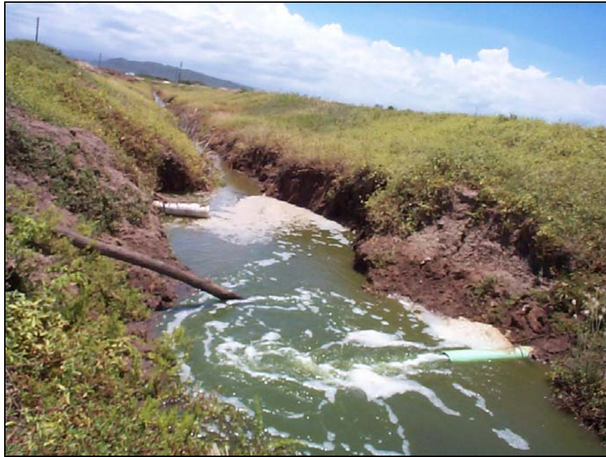
Plate 13. Typical erosion caused by pond effluents during draining of ponds.
