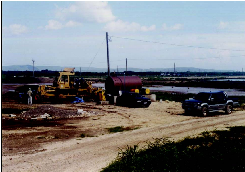
Plate 23. Fuel pump and storage tank facility under construction.
