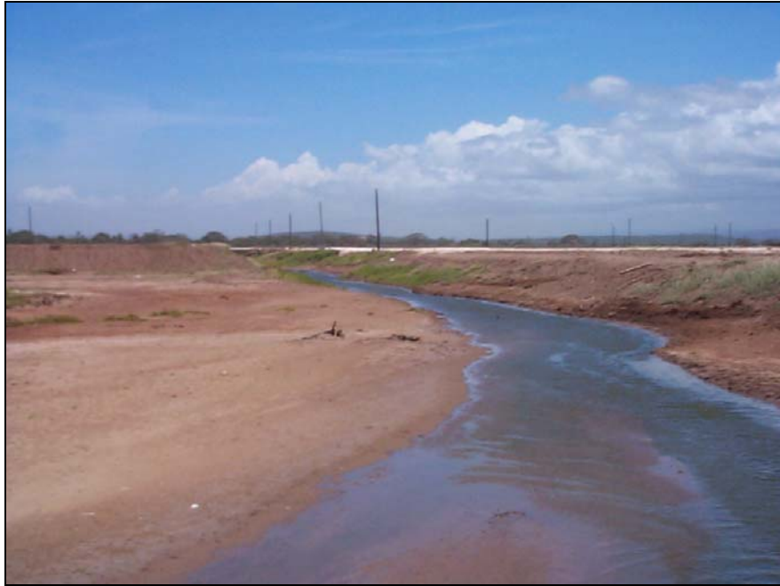
Plate 17. Storm water drain passing through farm emptying into 'artificial wetland' area.
