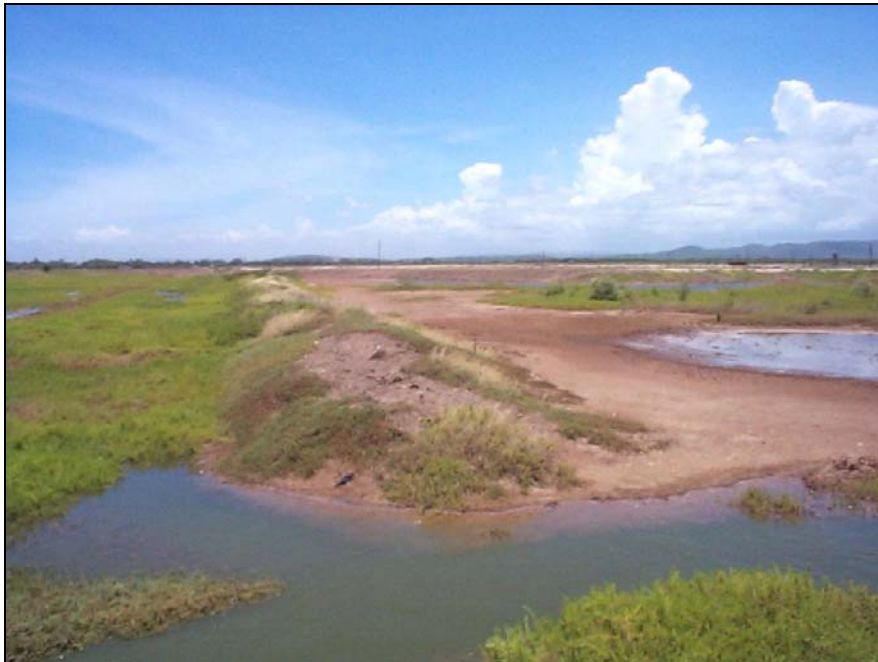
Plate 18. 'Artificial wetland' area showing flood containment berm.
