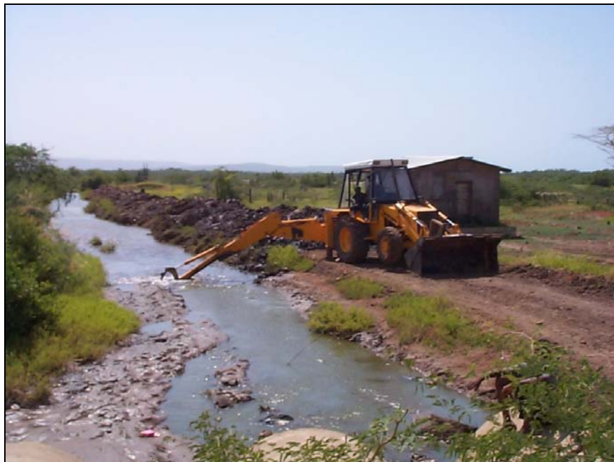
Plate 16. Clearing of silted drain leading to salina.
