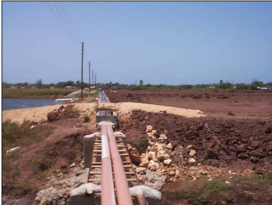
Plate 4. Water supply system to CMPL production ponds.
