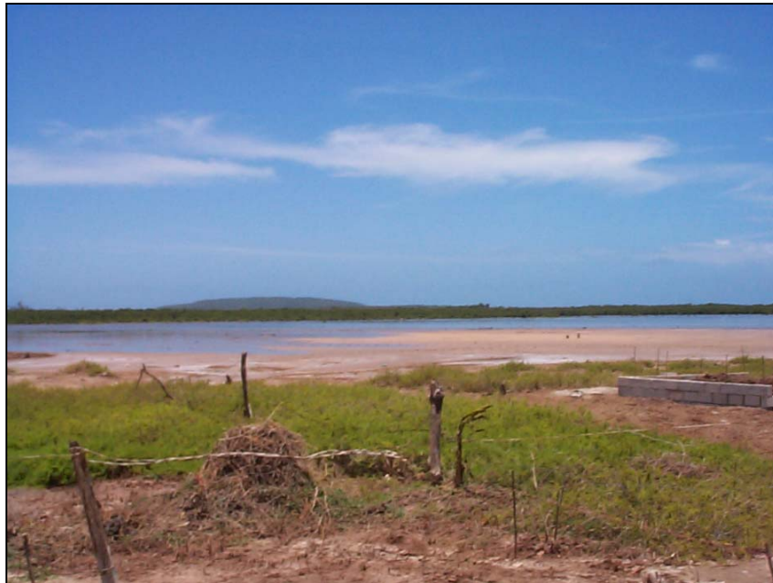
Plate 30. Foundation of house being built immediately adjacent to salina.
