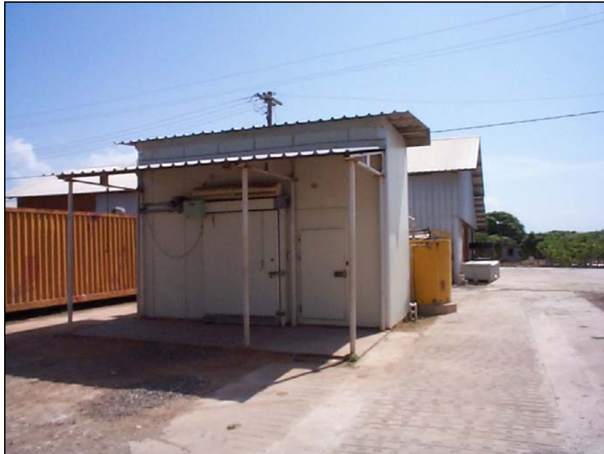
Plate 6. Existing processing and packaging facility at Brampton, St. Catherine.
