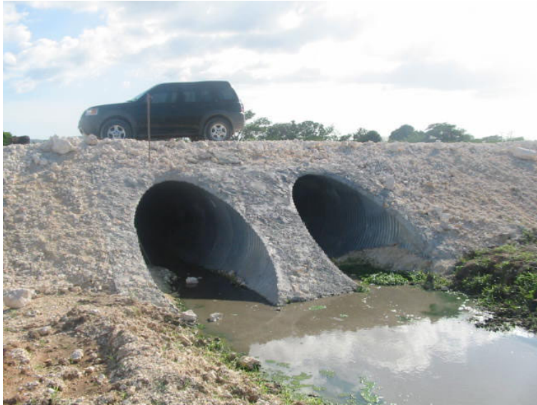
Plate 3 Central drain 2X4' culvert along H2K
