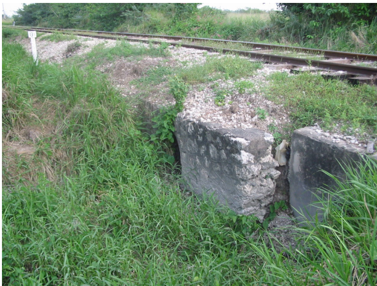
Plate 2 Central drain culvert along railway
