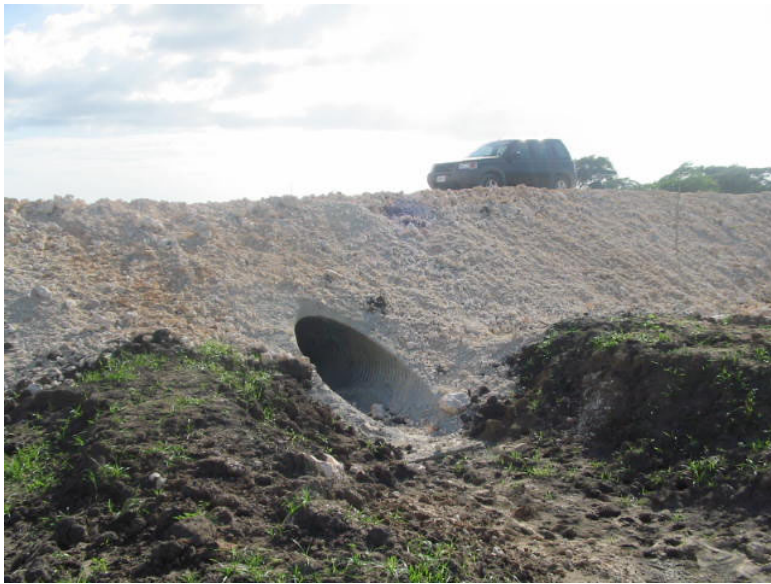
Plate 1 Eastern drain 4' culvert along H2K
