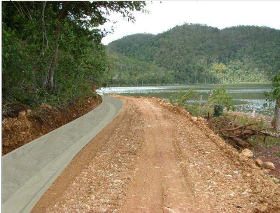
Figure 5: Illustration of the track and ditch
