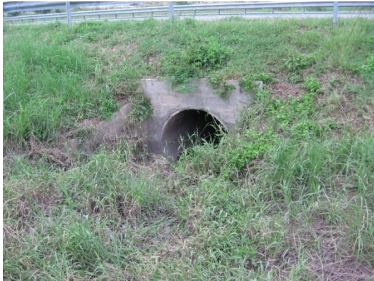
Photo 3 - 1.22m Dia. RC pipe below H2k
