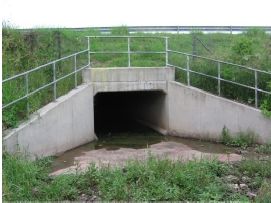
Photo 1 - 2.4mWide x 1.5mHt RC Box Culvert below H2k
