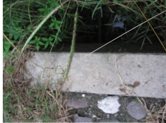
Photo 2 - 0.914m Dia. RC pipe culvert below H2k
