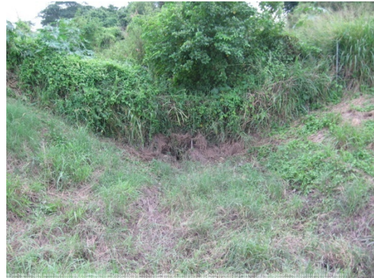
Photo 4 - Existing drain downstream of the 1.22m Dia. culvert
