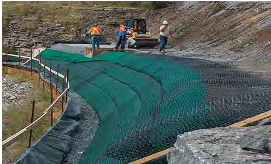
Plate 9.10 - Geogrids being placed on face of slope
