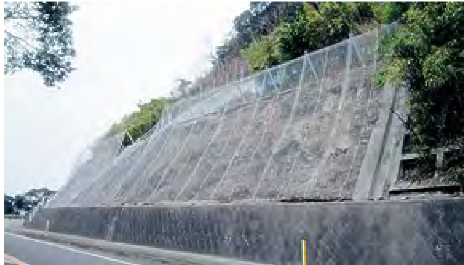
Plate 9.1 - Rockfall catchment fences being implemented
