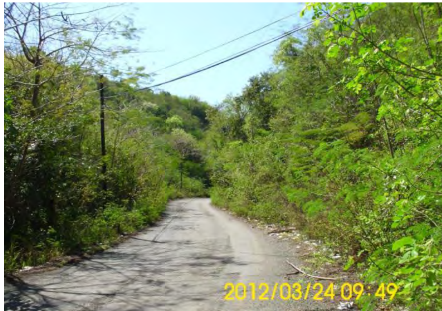
Plate 4.37 - Roadway through Location C, bordered on both sides by Leucaena leucocephala (Lead Tree) and Delonix regia (Poinciana) trees
