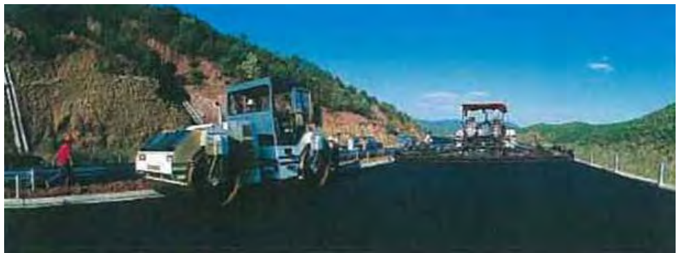
Plate 2.4 - Spreading and Compacting Asphalt Mixture (source CHEC)
