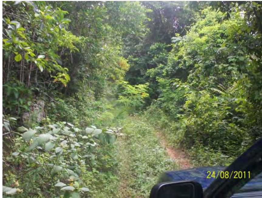
Plate 4.33 - Section of roadway along southern slopes of the St. Johns Red Hills towards Gibraltore
