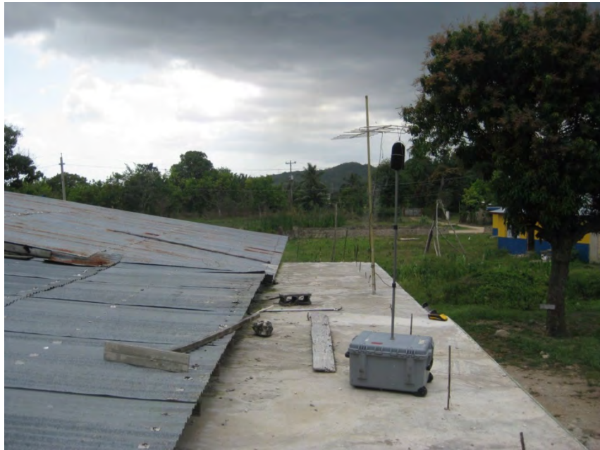
Plate 4.32 - Photo showing noise meter at Station N4 - Content
