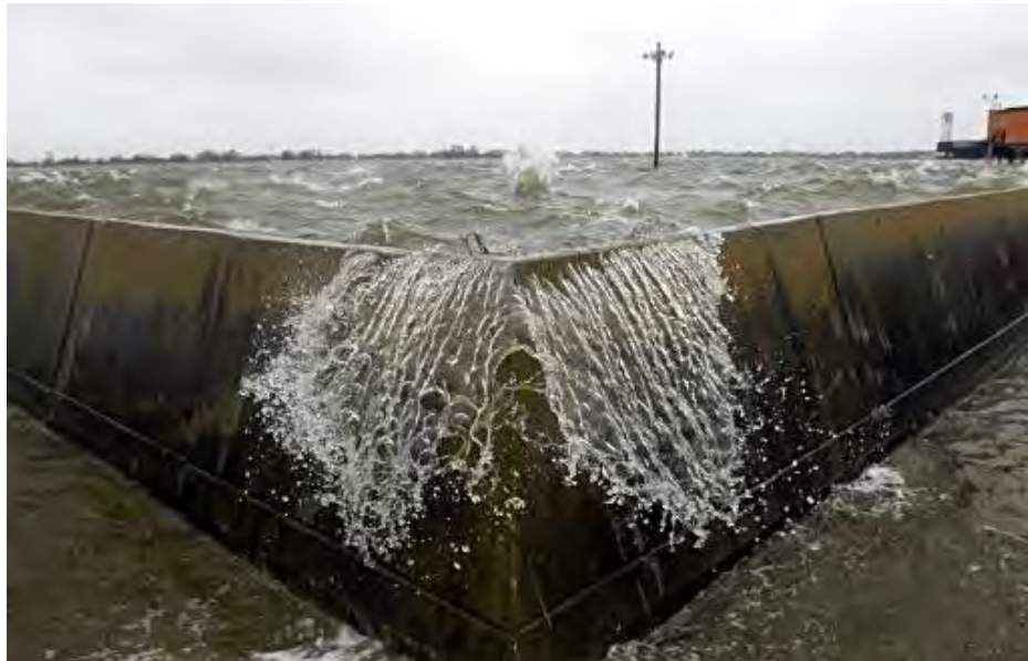
Plate 9.5 - Levee implemented in New Orleans during storm Gustav
