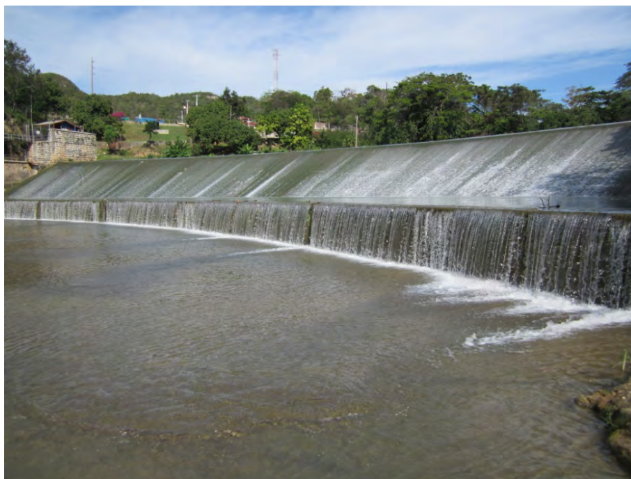
Plate 4.8 - Rio Cobre Dam situated downstream of the proposed alignment crossing
