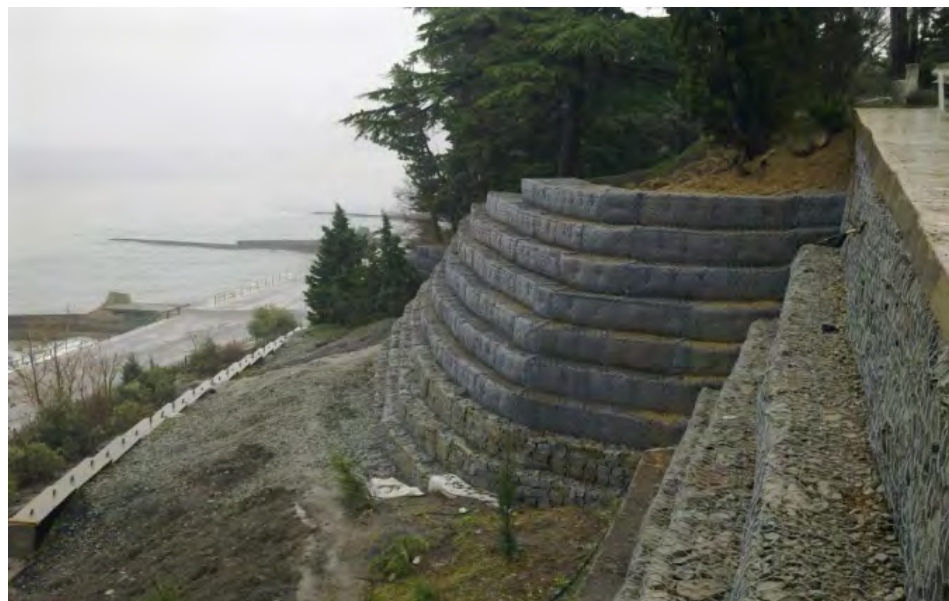
Plate 9.8 Gabion walls erected along face of steep slope
