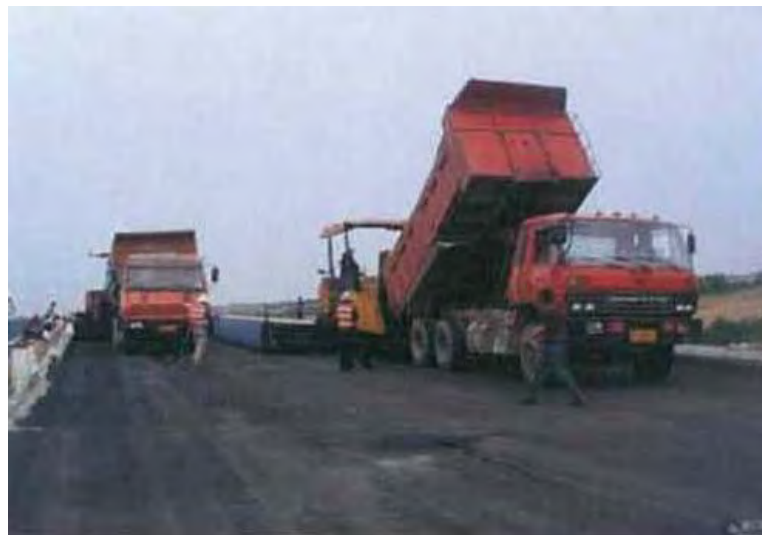
Plate 2.2 - Transportation of Asphalt Concrete (source CHEC)
