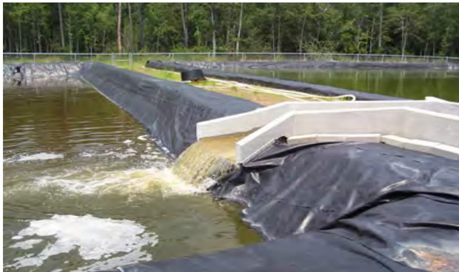
Plate 9.3 - Detention ponds used to reduce peak flows
