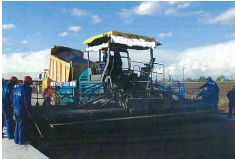
Plate 2.3 -Asphalt Concrete Spreading (source CHEC)
