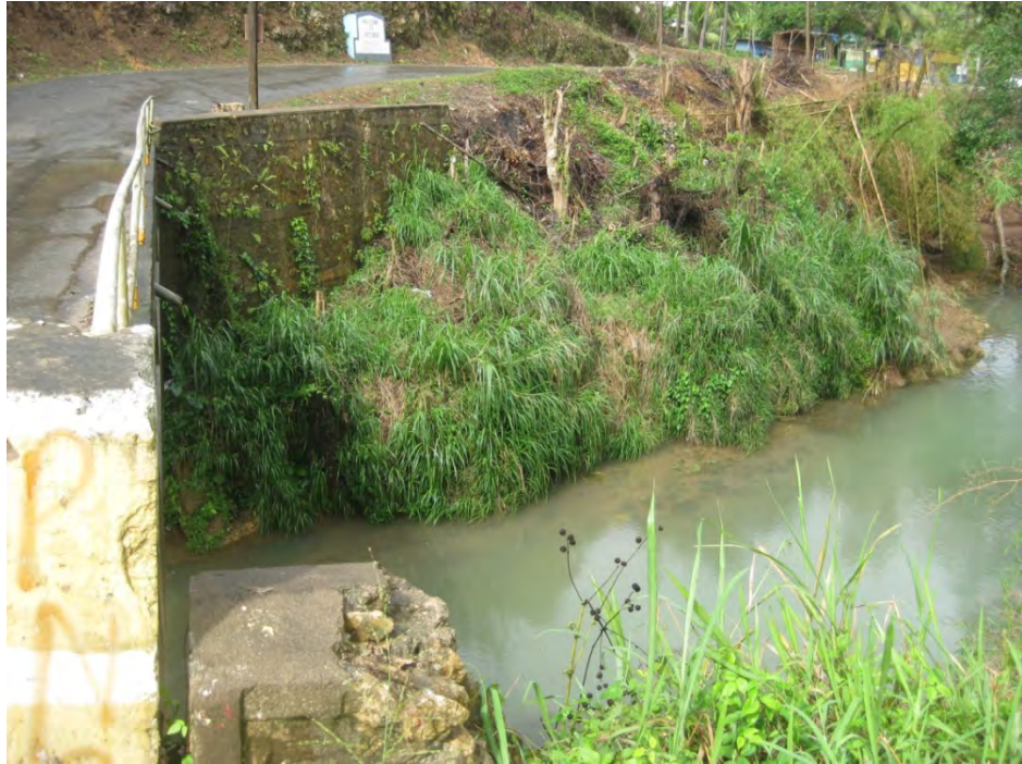
Plate 4.20 - Photo showing WQ7 – Rio Cobre by Victoria bridge
