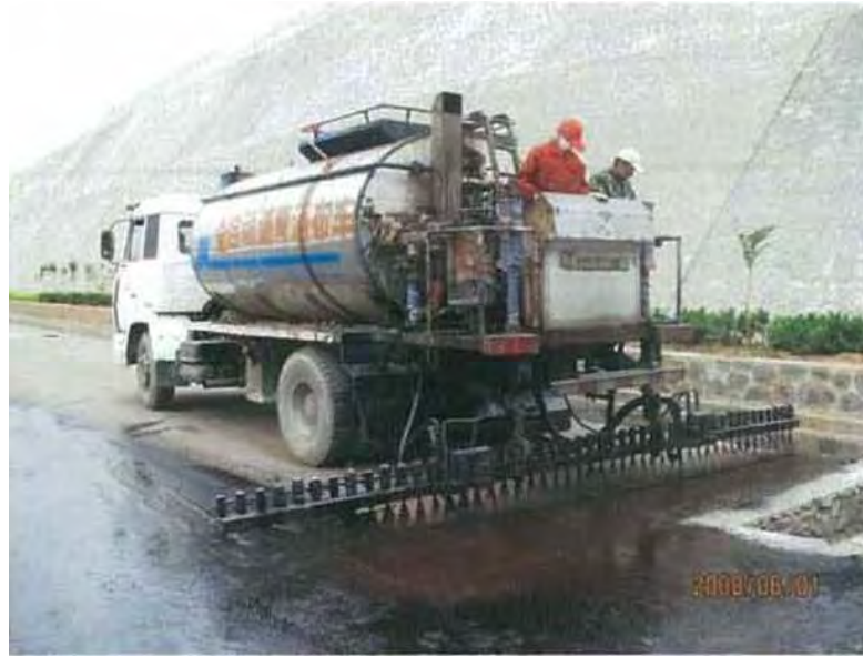
Plate 2.1 - Asphalt Pavement Construction (Spraying) (source CHEC)
