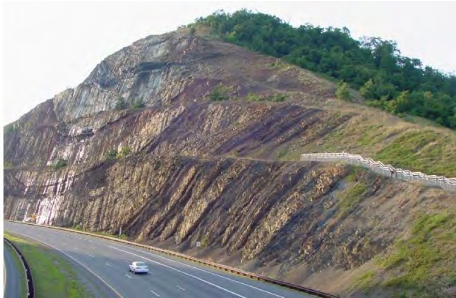
Plate 9.7 - Bench trail cut on face of steep slope
