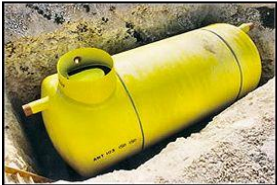
Plate 9-2 Filling station forecourt separator
