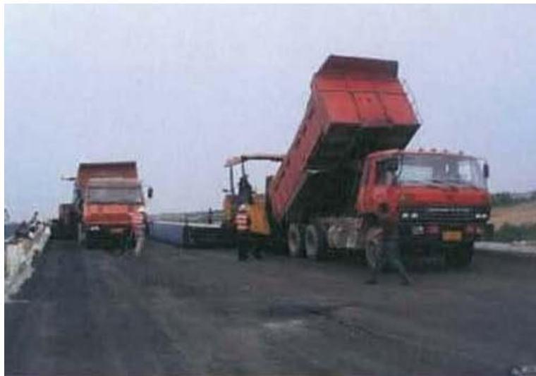
Plate 2-2 - Transportation of Asphalt Concrete (source CHEC)
