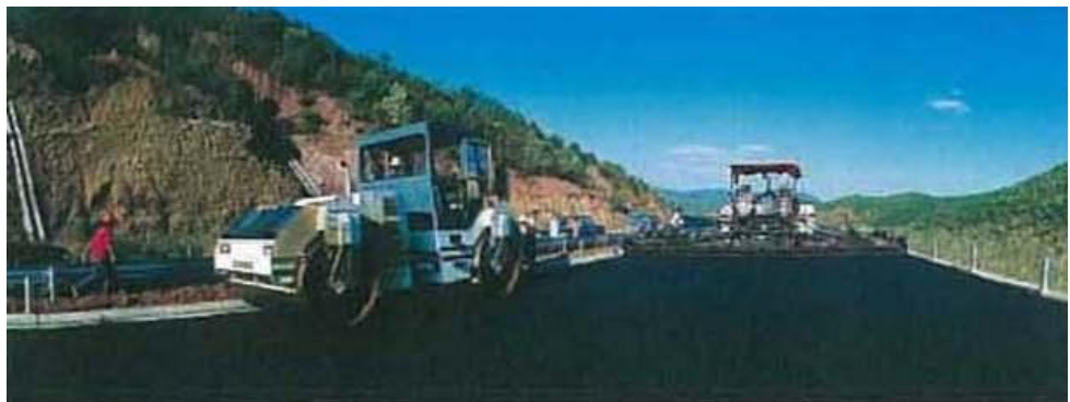
Plate 2-4 - Spreading and Compacting Asphalt Mixture (source CHEC)
