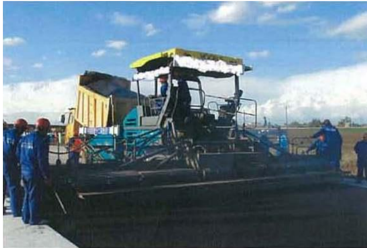
Plate 2-3 -Asphalt Concrete Spreading (source CHEC)
