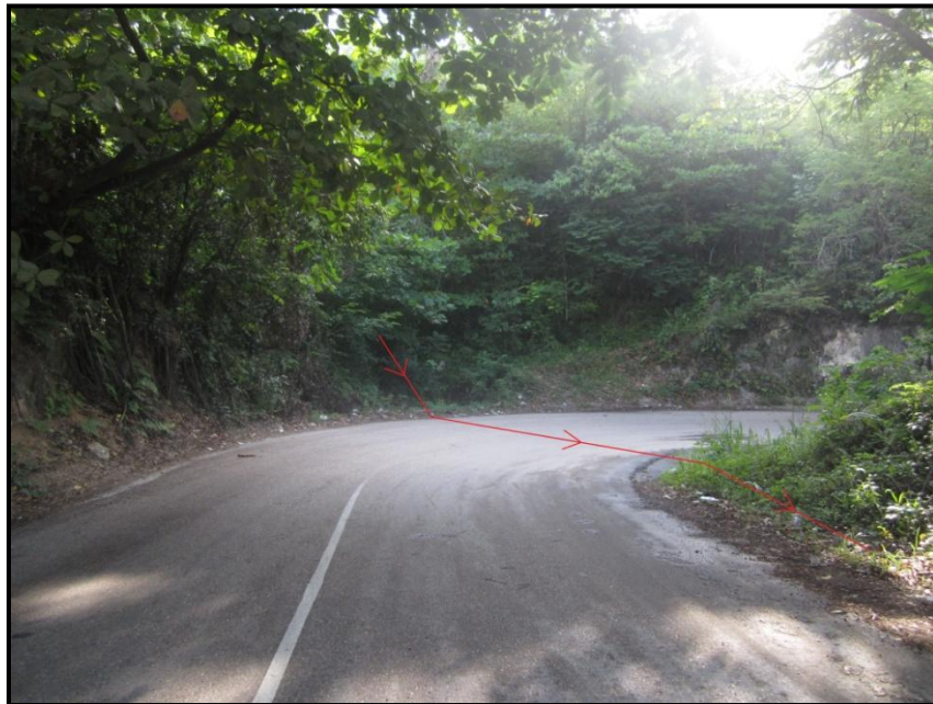
Plate 4-7 Illustrating the flow of Little River Tributary 2 under the existing road via pipe culvert.
