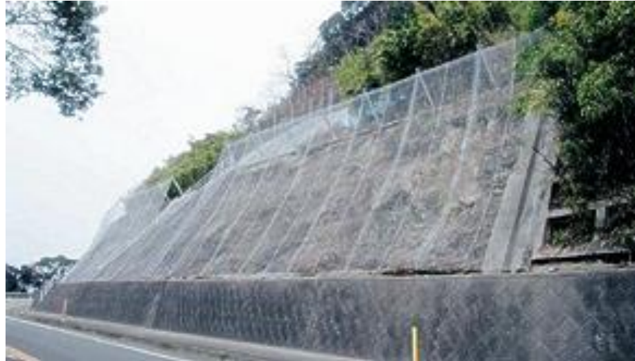
Plate 9-1 - Rockfall catchment fences being implemented
