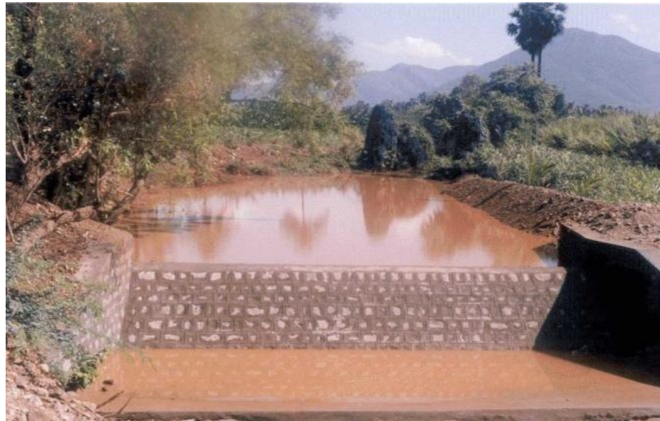
Plate 9-11 - An example of a check dam being used
