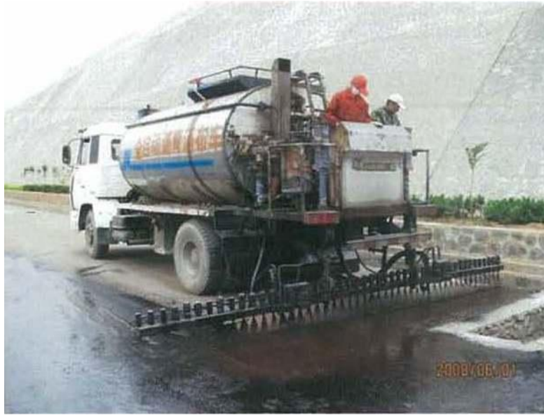
Plate 2-1 - Asphalt Pavement Construction (Spraying) (source CHEC)
