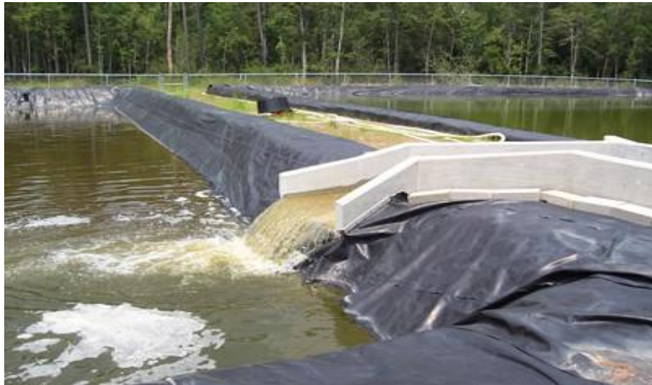
Plate 9-3 - Detention ponds used to reduce peak flows
