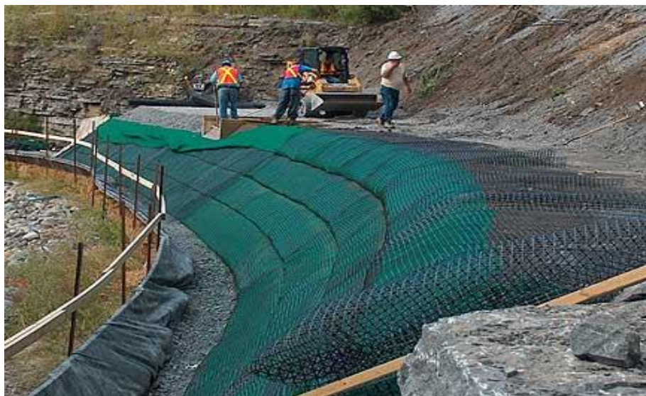
Plate 9-10 - Geogrids being placed on face of slope
