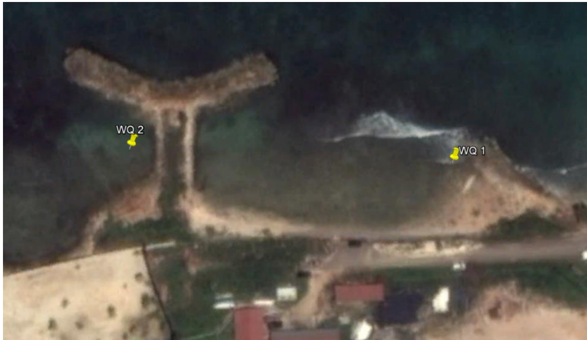
Figure 2.3 Location of water quality samples (WQ1 & WQ2) taken from the project area
