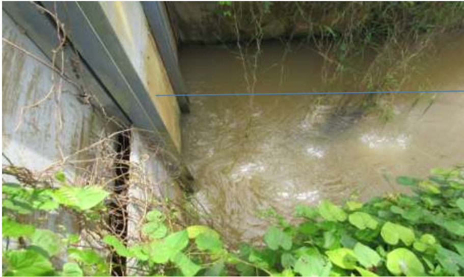
Figure 3:4 Sluice gates observed on the BR UM used to control flooding and irrigation purposes
