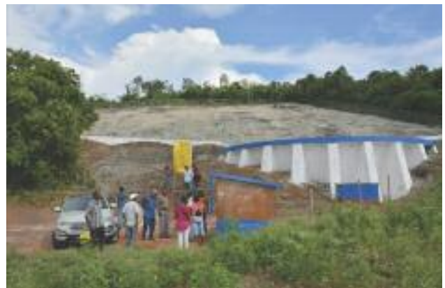
Rainwater Harvesting – Rose Hall, St. Elizabeth
