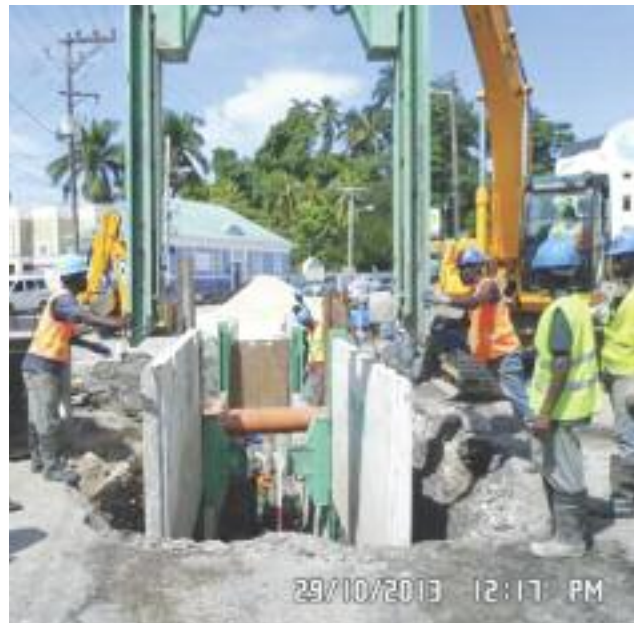
Sewer Works in progress, Fort George Street, Portland
