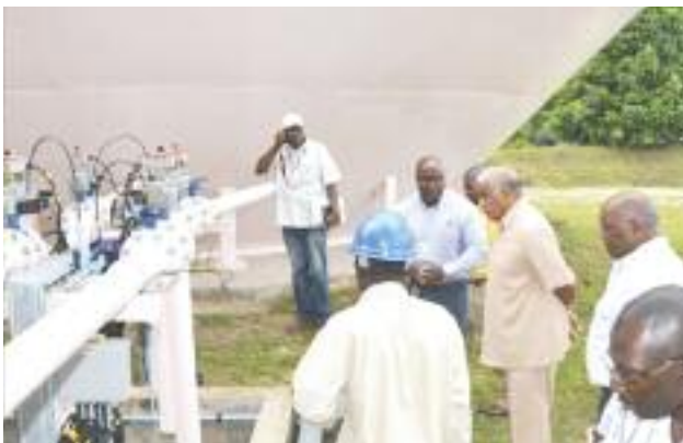
Commissioning of the Bogue Water Treatment Plant
