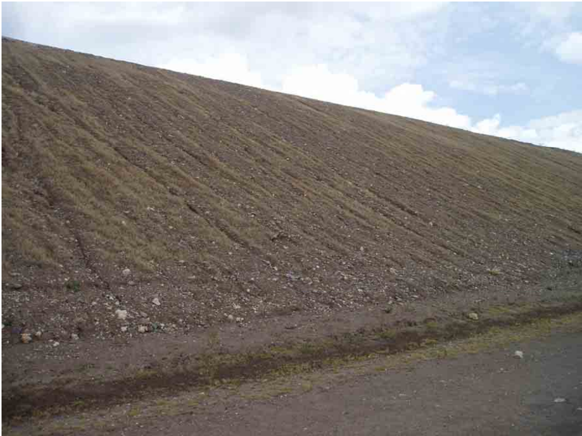
FIGURE 3-26: GRASS COVERING SLOPE OF DYKE OF RESIDUE DISPOSAL AREA.
