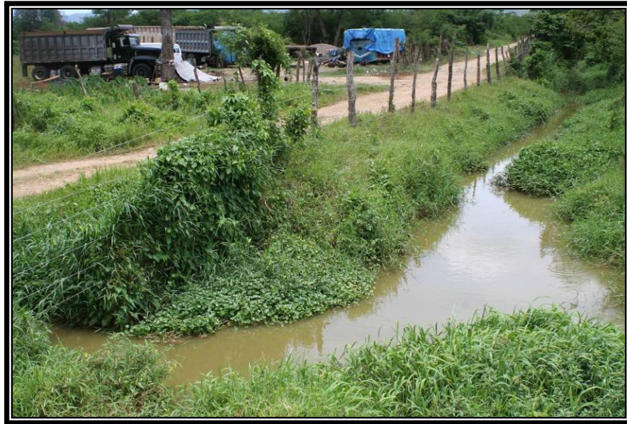
Plate 7.2: Looking south at approximately km 56+800 (May 04, 2007).
