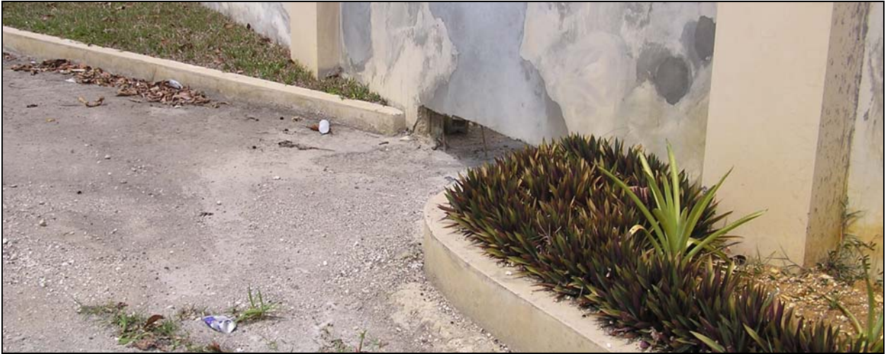
a/ Drain from main road to the site
