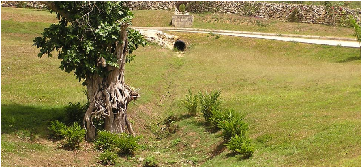
b/ Drain from Copse road to the site
