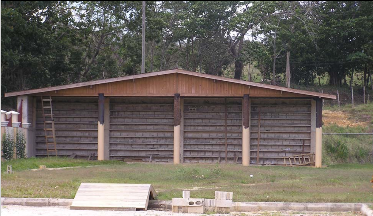
Figure 4 Structure on the South-Western Corner of the Property
