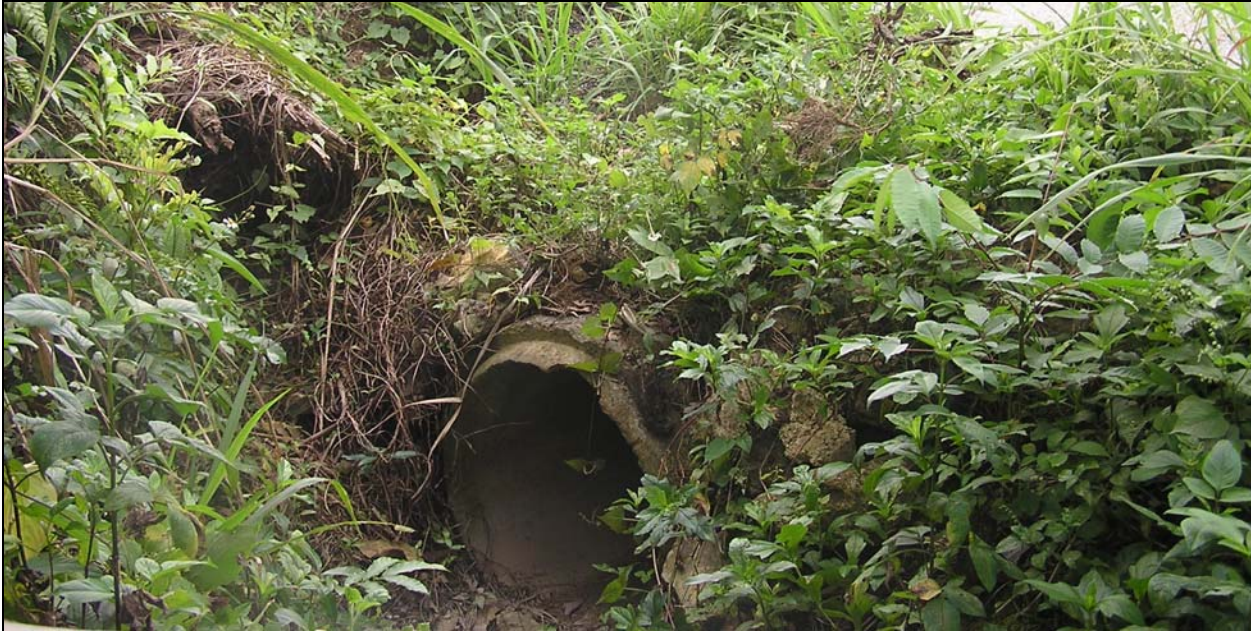
c/ Drain under main road.
