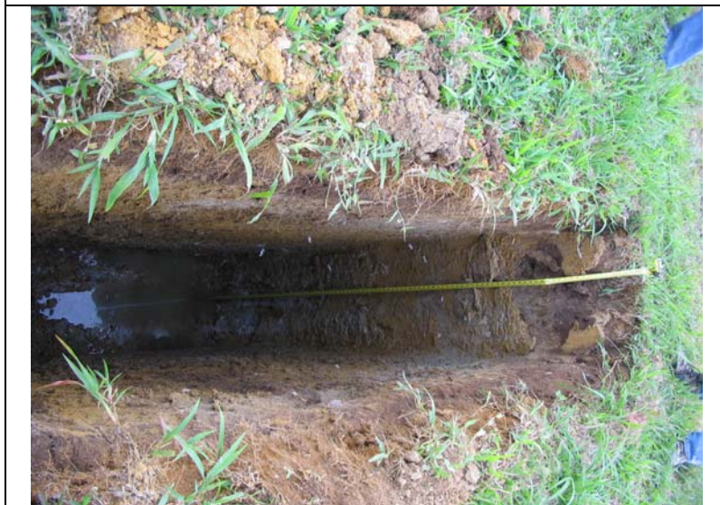
Figure A.14 Pit 7 groundwater inflow about 2.65 m
