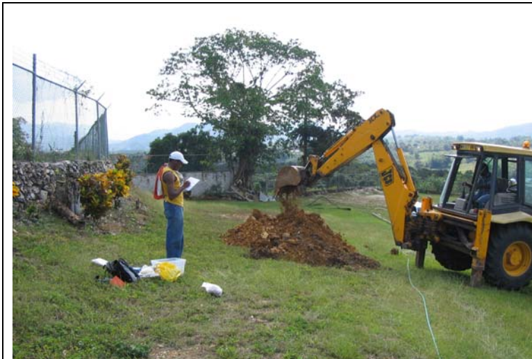
Figure A.4: Pit 2 Location adjacent to north-eastern boundary – gentle slopes
