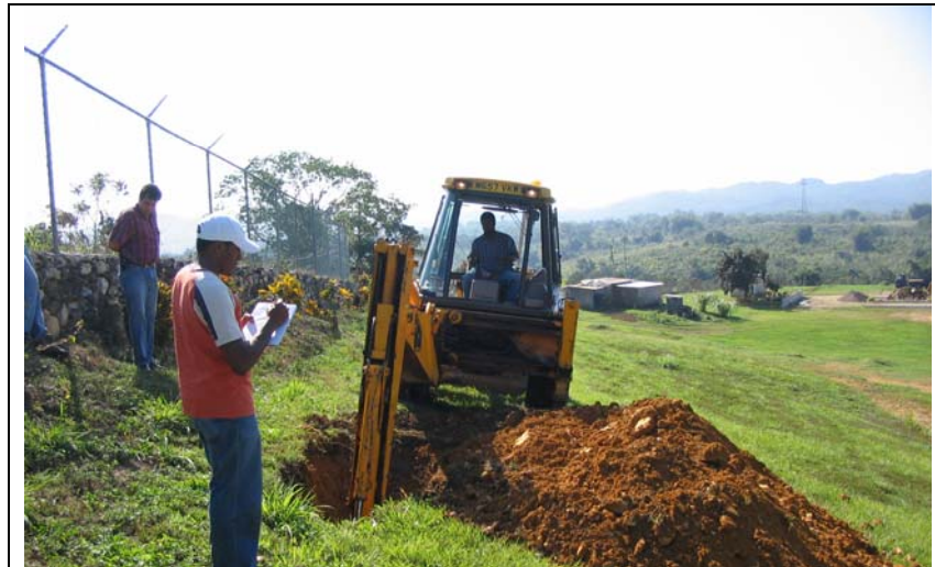
Figure A.1: Pit 1 Located at north-eastern corner
