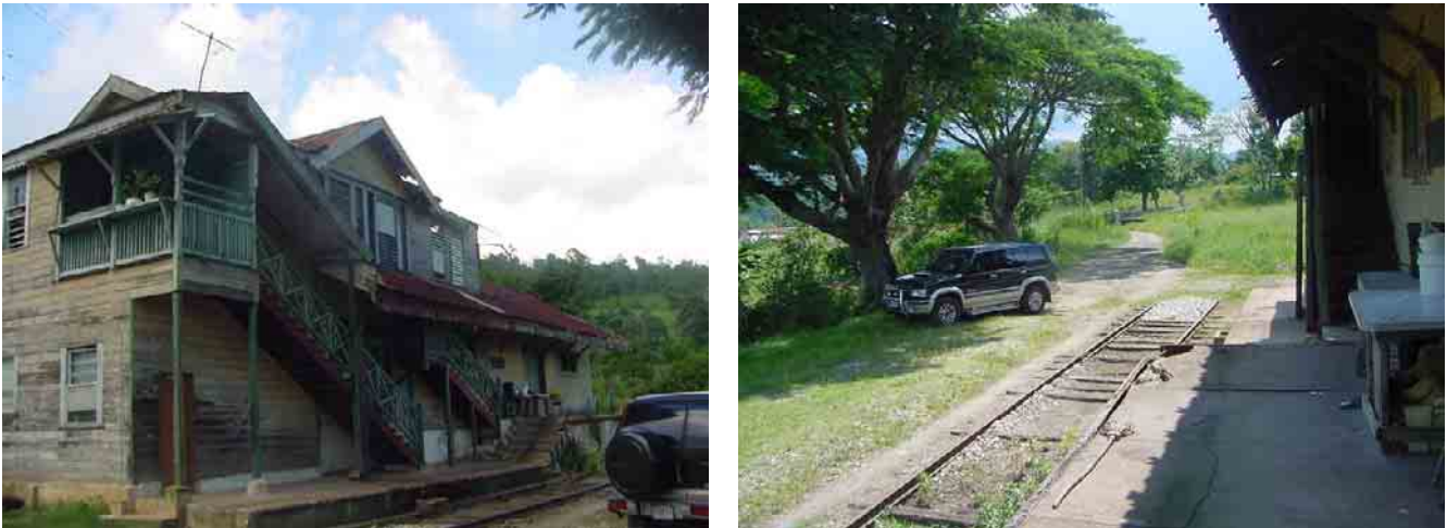
PLATE 1-1: MILE GULLY RAIL STATION (NOT IN OPERATION FOR PAST 20 YEARS)
