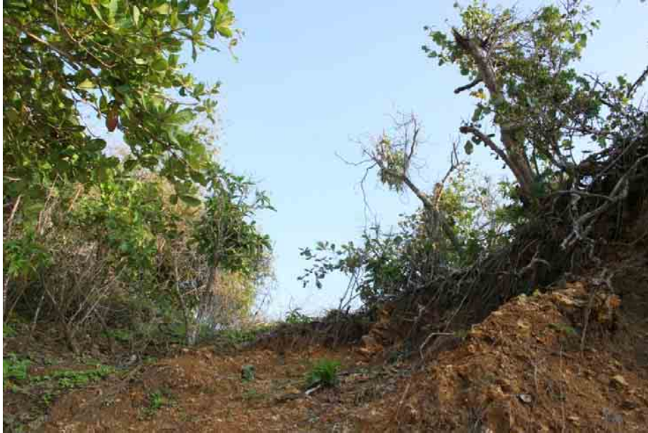
Photo 11: Erosion observed on the eastern promontory of the bay
