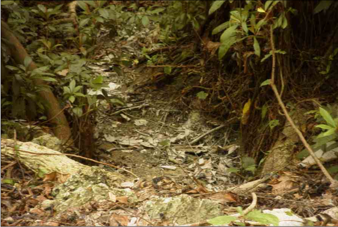
Photo 6.2 - Natural Gully showing evidence of hydraulic scouring (May 12, 2006)
